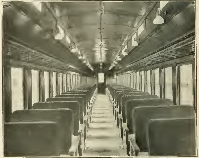
Interior of the New Haven Steel Coach
