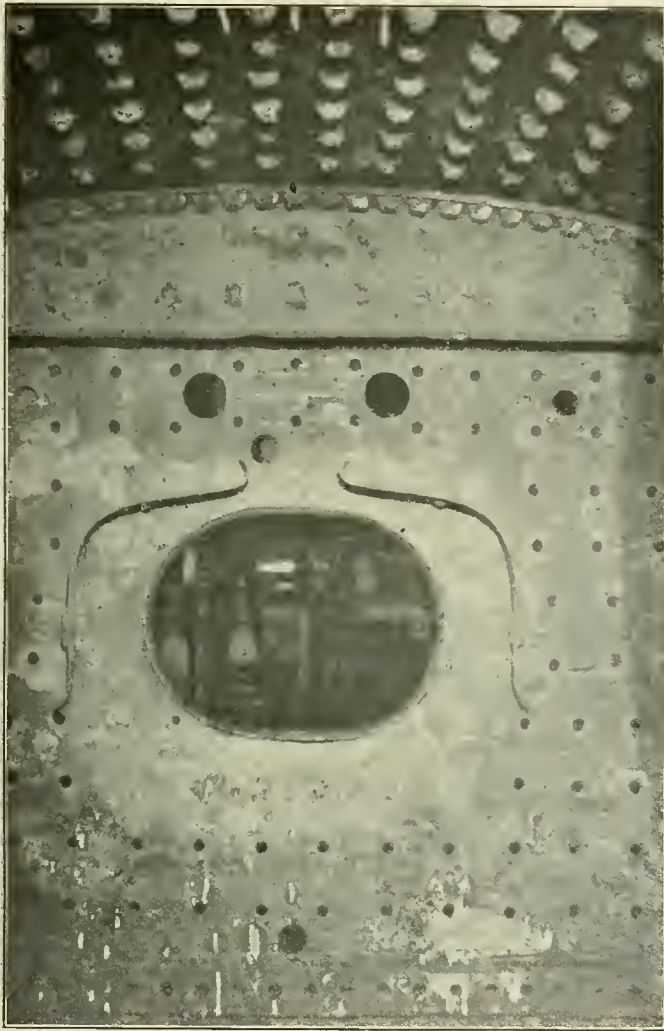
Fig. 5—Three-Fourths of Door Sheet Removed
