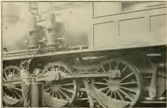
Burning Out Oil Deposits in Air Pumps
