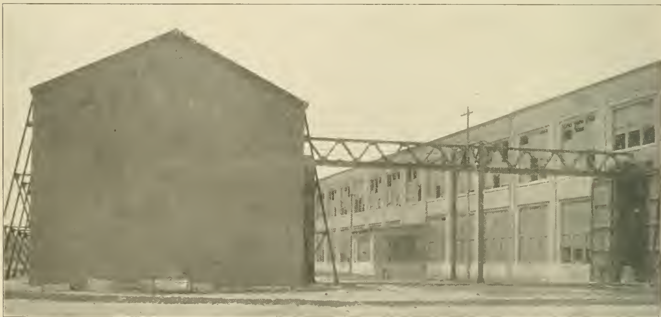
Tire Setting House and Monorail Hoist Runway from the Tire House to the Locomotive Shop
