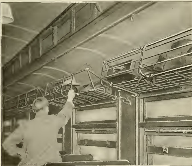
Safety Baggage Rack in Santa Fe Coaches
