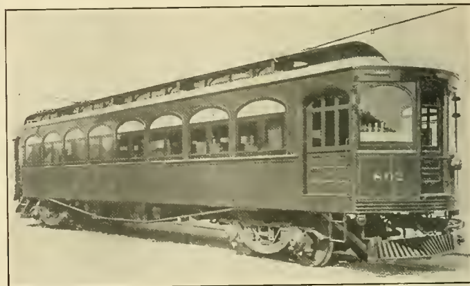
Heavy Interurban Car with Roller Bearings
