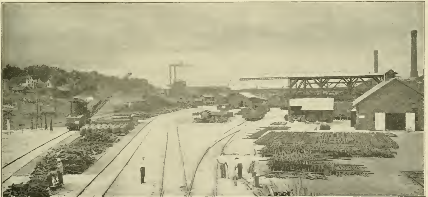
General View of Scrap Yard and Reclamation Plant
