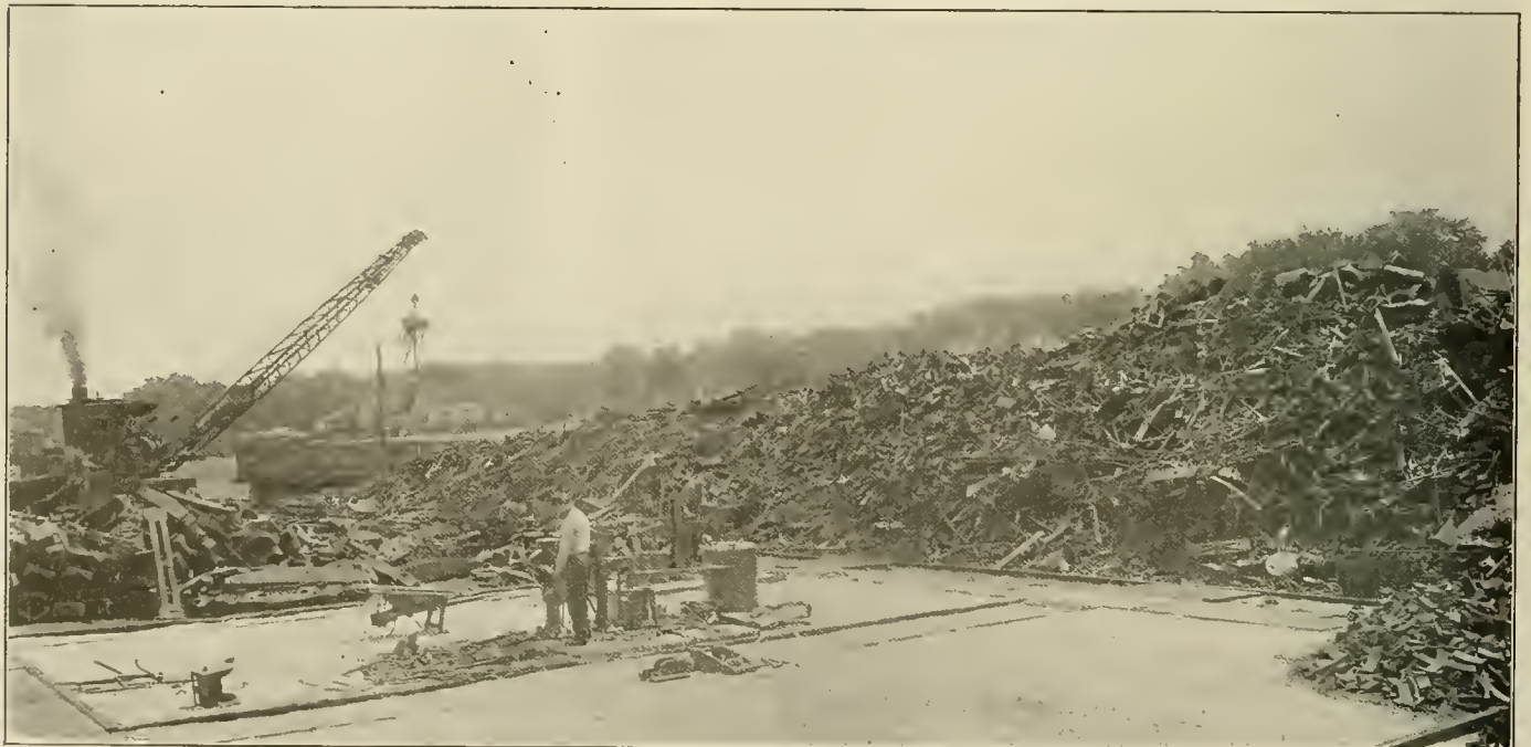
Unloading Scrap With a Three-Ton Hoist Equipped With an Electric Magnet
