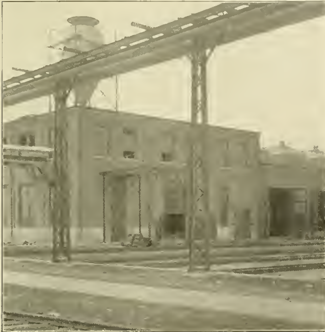
Pipe Supports, North End of Passenger Car Shop
