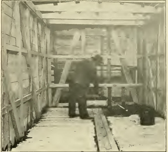
Applying Hot Asphaltum to the Car Floor
