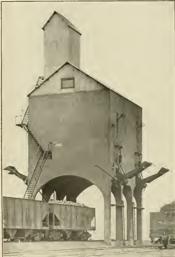
Reinforced Concrete Coaling Station at Blue Island, Ill.
