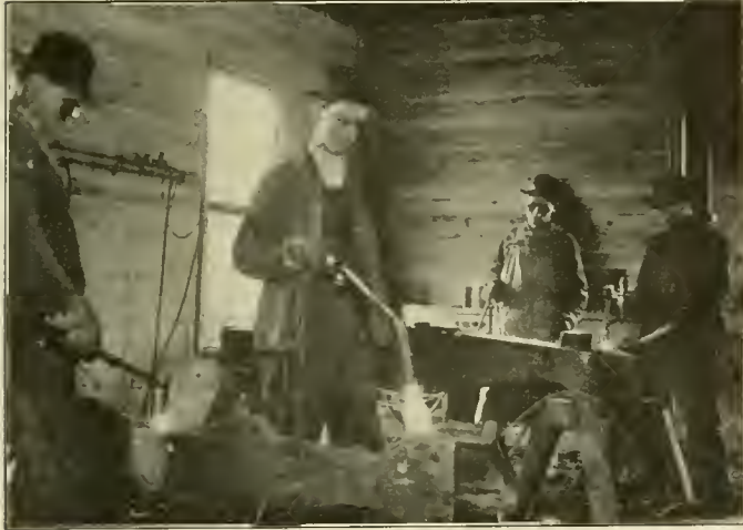
Welding Car Bolsters with the Oxy-Acetylene Process
