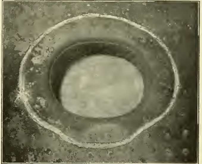
A Fire Door Hole Patch Welded in by Electricity
