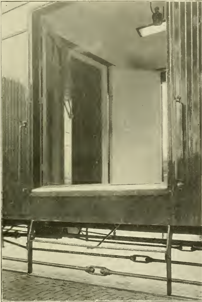
Side Doors and Bulkhead of Baltimore & Ohio Milk Refrigerator Car
