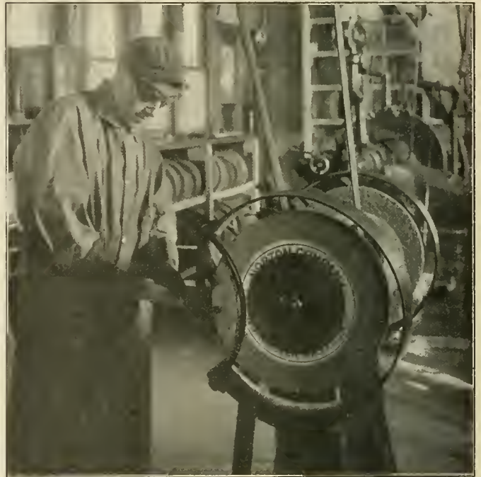
Protection Hood, Leather Spark Brush, Gloves, Goggles and Proper Rest Adjustment
