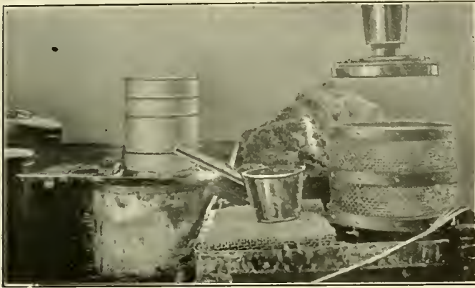
Equipment Used in Reclaiming Journal Box Packing
