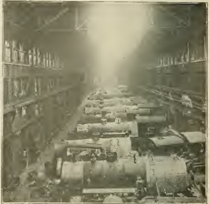
Lake Shore & Michigan Southern Erecting Shop at Collinwood, Ohio, Lighted with Cooper-Hewitt Quartz Lamps
