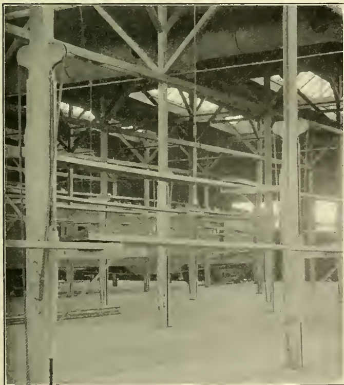
Fig. 1—Adjustable Staging for Painting Cars
