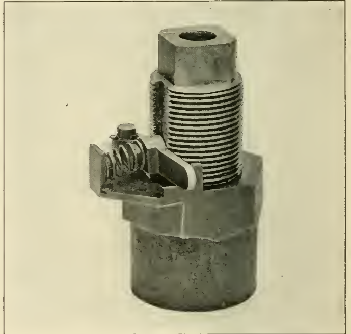
Grease Plug Fitted with a Locking Device
