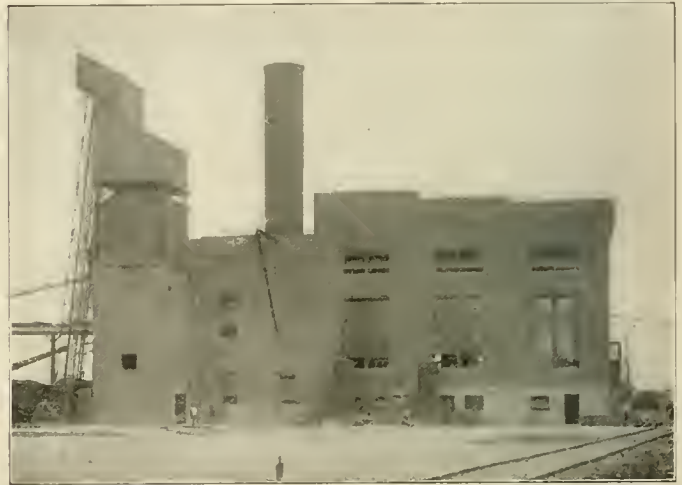
Power House, Showing the Coal Tower
