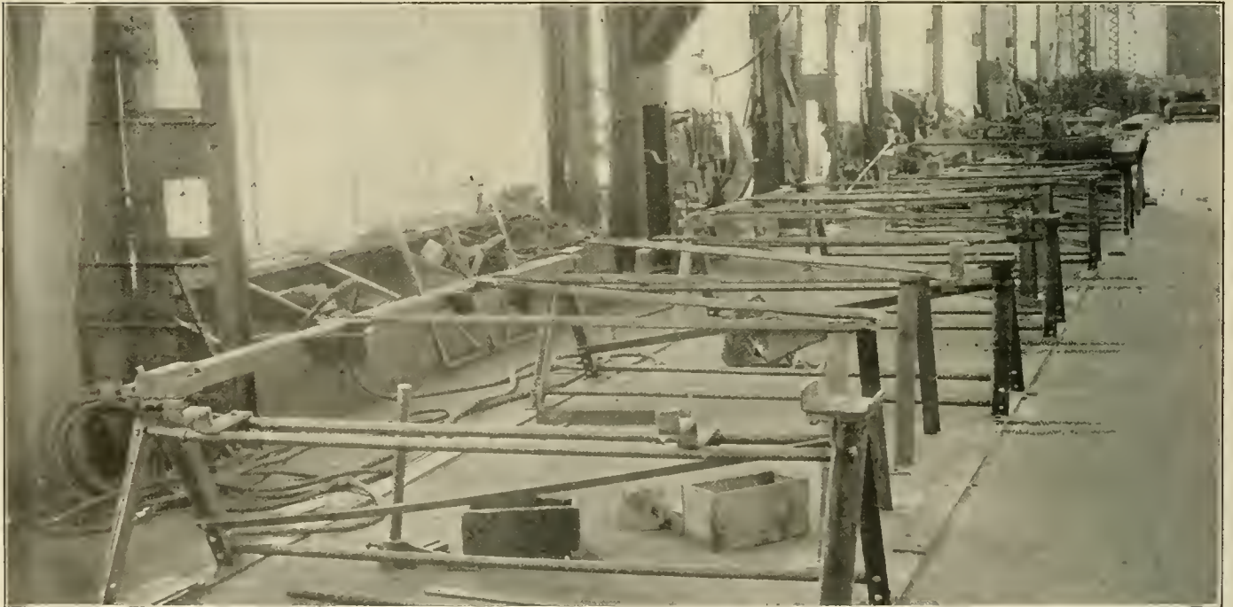
Template for Setting Up Side Framing; the Pockets are for Holding Tools
