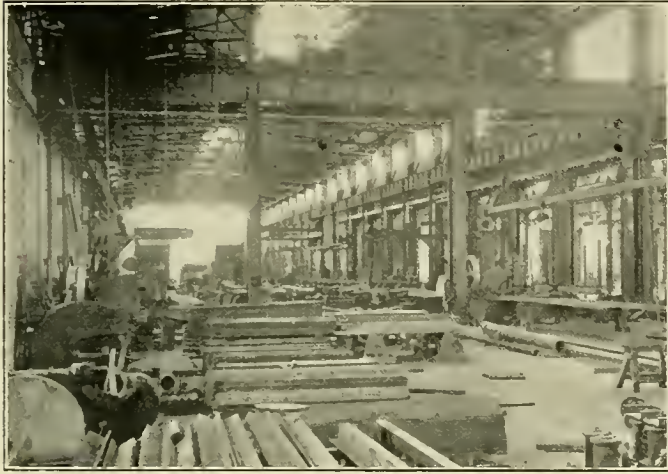
General View of the Freight Car Erecting Floor
