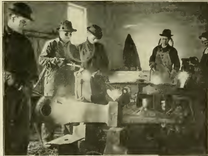
Repairing Car Bolsters, a Journal Box and a Coupler with Oxy-Acetylene
