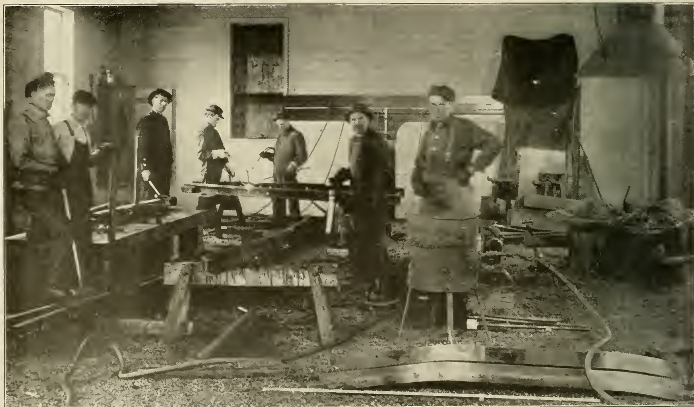
The Shop in Which Frogs and Switches Are Repaired and Reassembled
