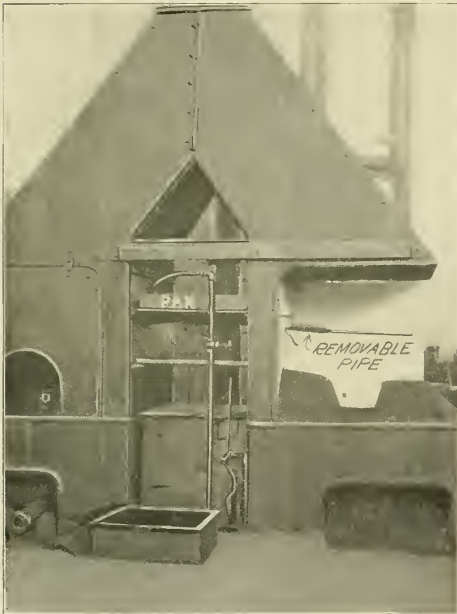
Safety Device for Quenching Forge Fires
