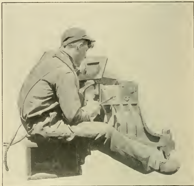
Surface Built Up on a Truck Casting
