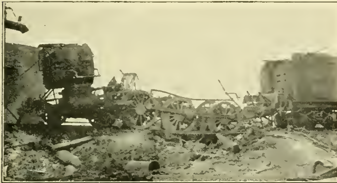
Result of a Boiler Explosion Caused by Defective Crown Bar Braces
