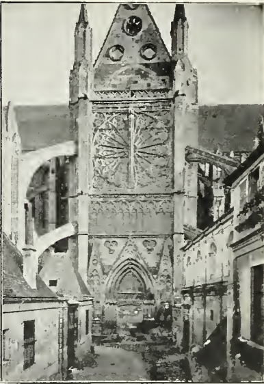
FIG. 104.—TOURS CATHEDRAL. (The Flying Buttress.)
