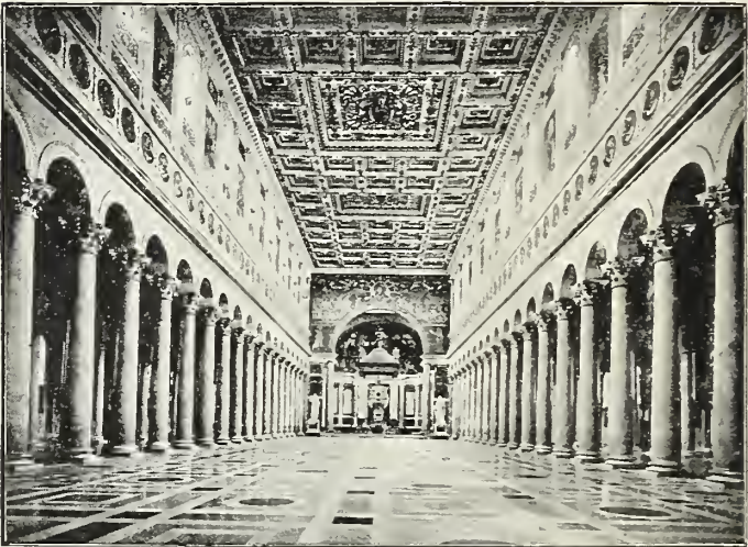
FIG. 51.—BASILICA OF ST. PAUL. Rome. Rebuilt 1828. Old Church, Fourth Century.
