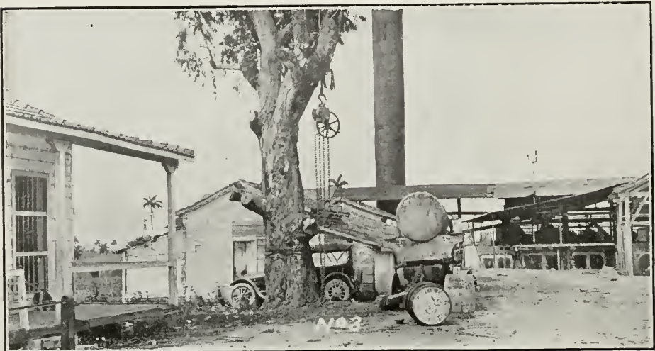
Boiler House of Small Cuban Central.
