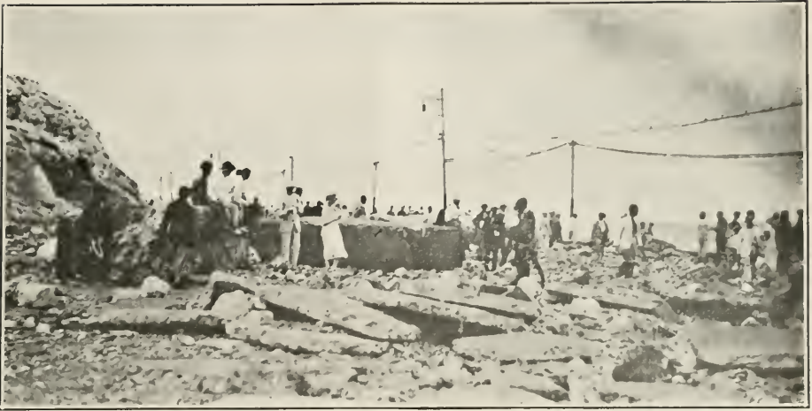
View of the driveway connecting Havana and Vedado, showing huge portions of the new concrete seawall, broken up by the waves during the storm. These ruins of the seawall were carried entirely across the new boulevard now being constructed along the seawall, then over the double street-car tracks and were finally deposited in the middle of the roadway at the foot of Santa Clara Battery, as shown. The blocks were so large and heavy that it was necessary to blast them into smaller sections for removal. The rough slabs in the foreground are pieces of the concrete base of the new boulevard mentioned above. (Photo by Harris Bros., Havana.)
