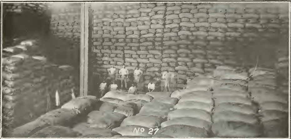
Sugar in Warehouse, Cunagua.
