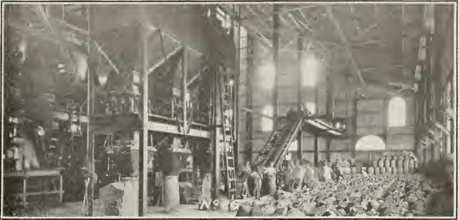
Automatic Bagging and Weighing Scales, Cunagua.
