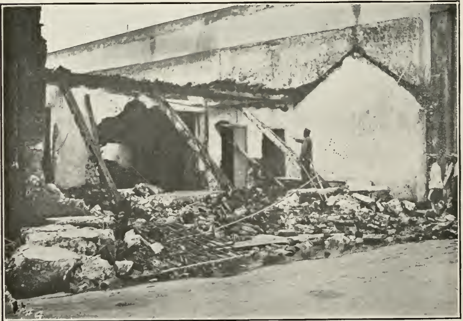
Small house on Marina Street, completely wrecked by the waves during the storm. The street itself is flooded, as may be seen by the water in the foreground. Practically all the houses on this street, which fronts the sea, were rendered uninhabitable. In many cases where the walls of the houses withstood the force of the waves, the door and window frames were completely torn from their places by the tremendous force of the water. (Photo by Harris Bros., Havana.)
