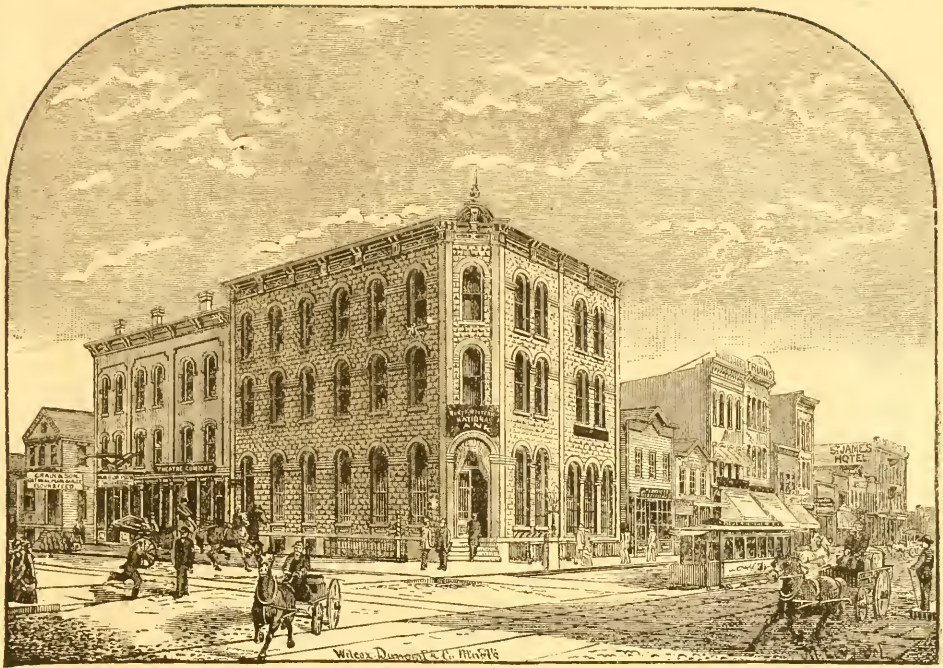
SOUTHEAST CORNER WASHINGTON AVENUE AND FIRST AVENUE SOUTH.
