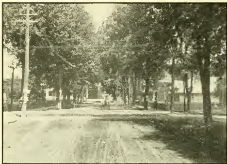
Bell & LeClere, Photo. VIRGINIA, NORTH ACROSS WILLIAMS.
