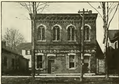
Bell & LeClere, Photo. THE WATERLOO OBSERVER BUILDING.
