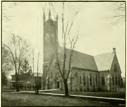
Bell & LeClere, Photo. ST. MARY'S CATHOLIC CHURCH.
