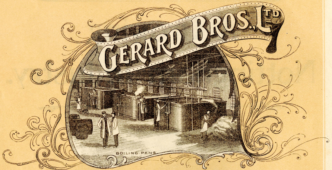
View showing three of the ten Boiling Pans. These are at a height of 30-feet from the ground level, and work on the latest gravity system, thereby saving all hand labour.
