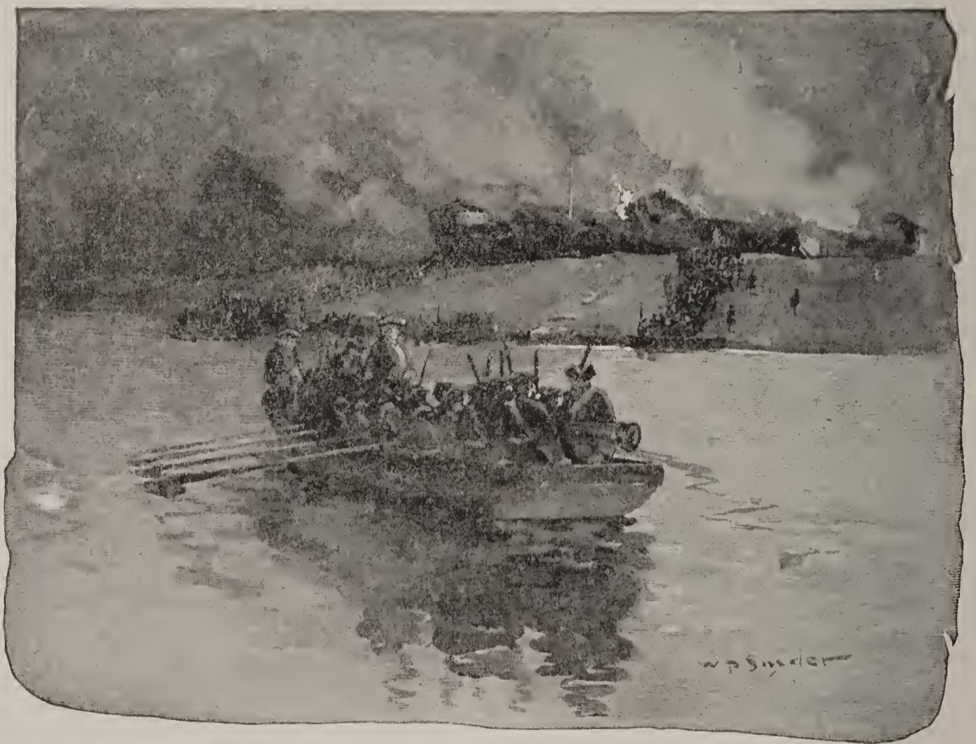
EVACUATION OF FORT DU QUESNE
