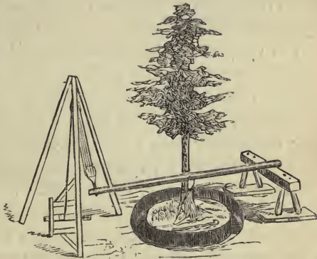
Apparatus for removing large trees.
