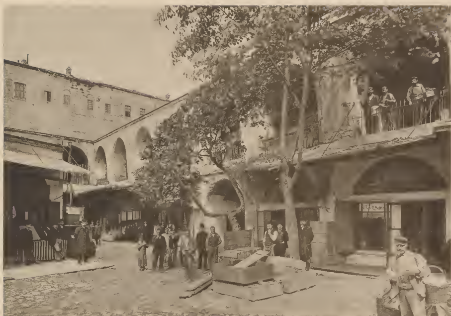
13. COURTYARD OF ÇOFNELI'S BUREAU
