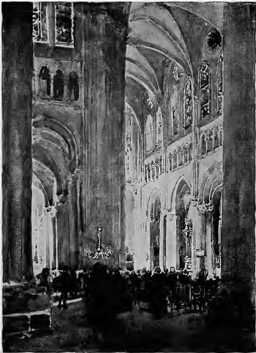
LOOKING INTO THE NORTH TRANSEPT FROM THE NAVE
