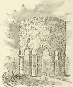
Tower at Newport.
