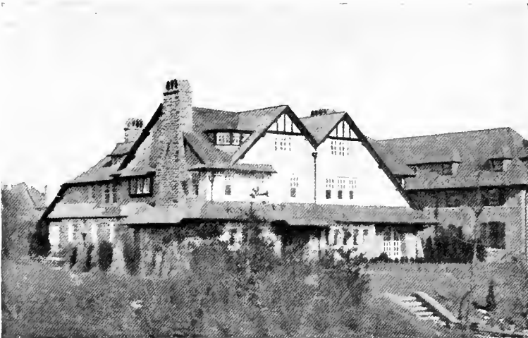
An interesting combination of stucco with half-timber work in the gable ends to avoid monotony. The Germantown hood extending over the first-story windows is a purely American feature
