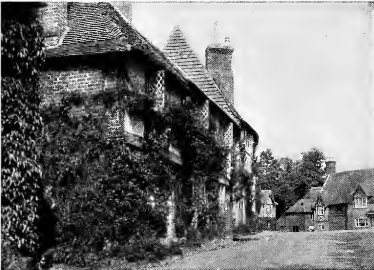
An example of the old English work where the walls are partly of brick and partly of half-timber work. Much of the charm in these English cottages is due to the mellowing influence of time
