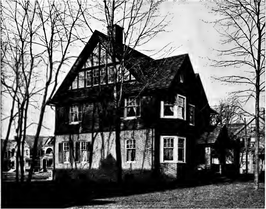
The Flemish bond brickwork, dark-stained shingles, the plaster-and-timber gable ends and the white trim of the windows, give a broad variety of materials that needs careful handling to be effective
