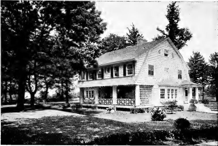
The second floor is made larger than the first by carrying the roof and long dormer out over the side porch
