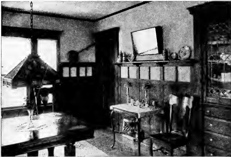
Stained cypress has been used effectively for the wood trim and the wainscotting, with its upper panels matching the tinted plaster
