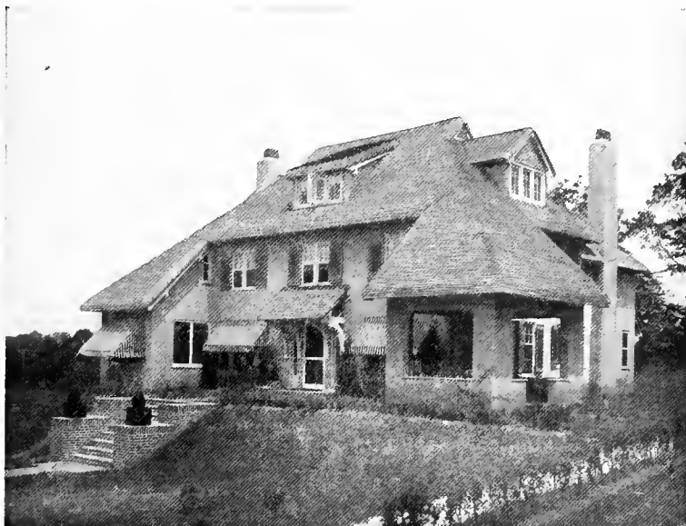
Although pleasing roof lines are obtained by use of shingles laid to imitate thatch, the cost of materials and labor is greatly increased
