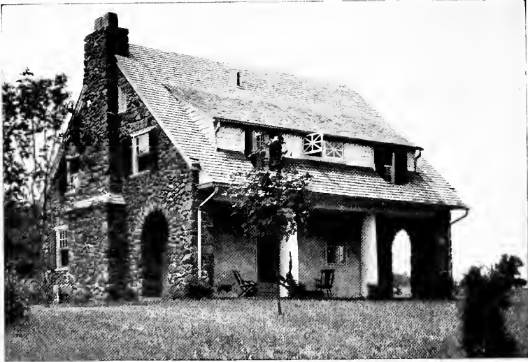
Where stone is used, a wall of cobbles is the most economical. Here only the end walls are stone; the rest, covered by the projecting roof, is of stucco over a frame wall
