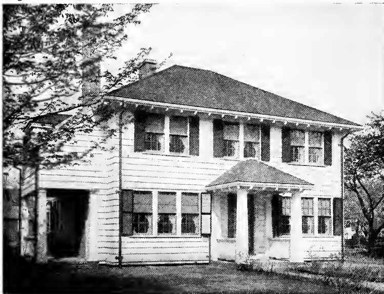
A painted clapboard house costs about thirty cents per square foot of surface. On side walls painted boards are more enduring than stone or shingles
