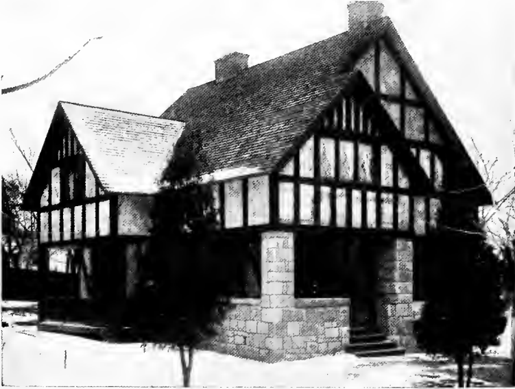
Half-timbering increases the cost of stucco on lath five cents a square foot. The stone foundation here is very expensive because of the carefully trimmed stone, and at the same time is less attractive
