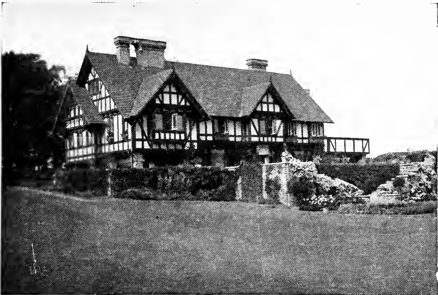
The English half-timber house as usually built in this country is merely a plaster house covered with wooden strips in a pattern. Here, however, the timbers are a structural part of the wall
