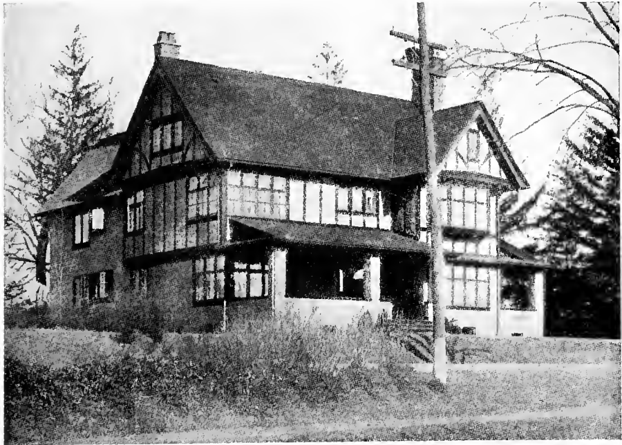
The common fault of overdoing the intricacy of the half-timber paneling has been carefully avoided
