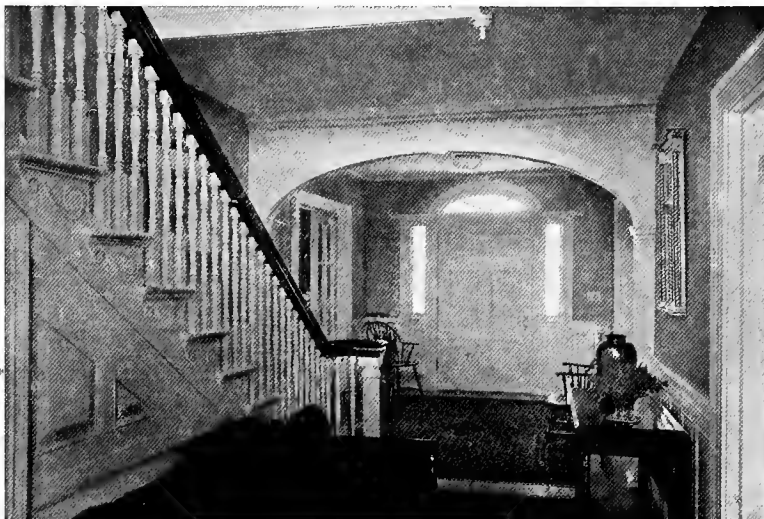
A view through the hall from the veranda end towards the north entrance door, showing the faithful Colonial detail of steps and balusters
