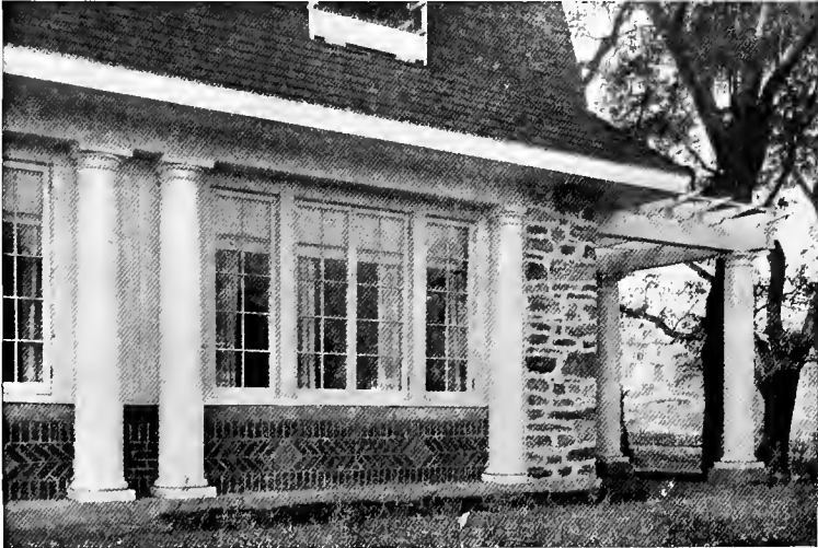
A curtain wall of brick and frame, between the heavy stone piers, gives the house a feature that is distinctly unique
