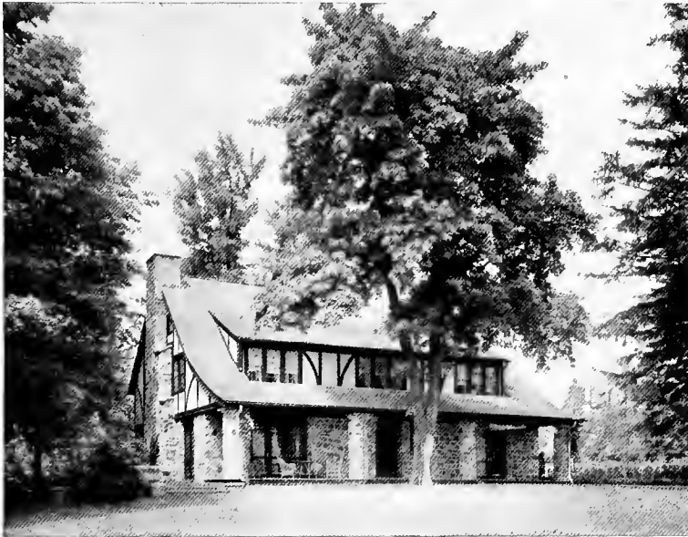
A country home at Pleasantville, N. Y. There is an interesting and unusual use of stonework in the circular columns supporting the wide overhang
