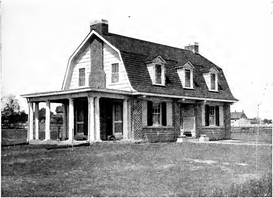
Mr. Flagg's cottage is an excellent example of how the very smallest country or suburban home that is really livable can be made attractive. The use of the heavy brick piers at the corners, with an unusual pattern of brickwork filling below the windows, and stucco walls above, makes the house particularly well worth studying.
