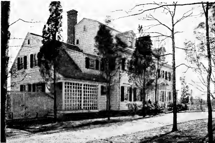
Like its New England prototypes, the house has its service end developed as a low wing. The laundry yard is enclosed by the lattice fence at the left
