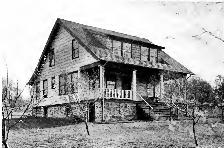
Wide boards are laid up horizontally like clapboards on the wood frame over the underpinning of local stone
