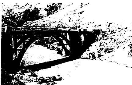
FIGURE 3. Masonry arch bridge over Mania river between Ambatofinandrahana and Ambositra (U/OU)
