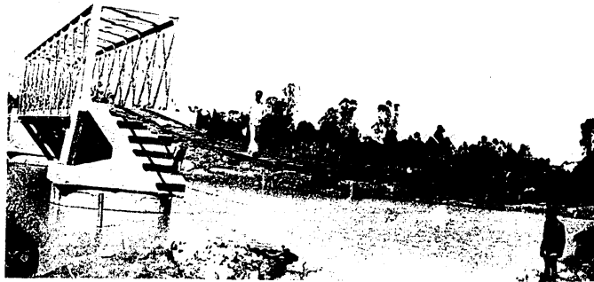
FIGURE 1. Damage to Iankana river bridge on the Moramanga-Ambatosoratra line caused by a recent cyclone (U/OU)
