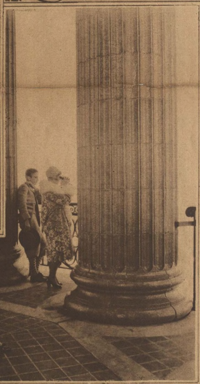
Detail of observation tower.
