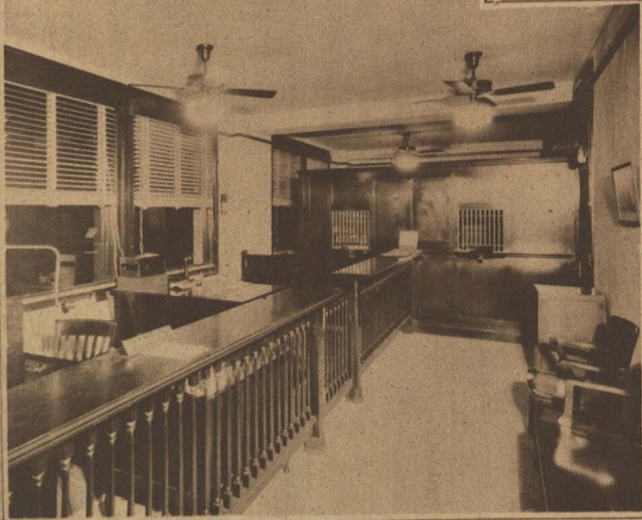
Partial view of lobby in offices of C. A. Bryan Real Estate Corporation on the eleventh floor.
