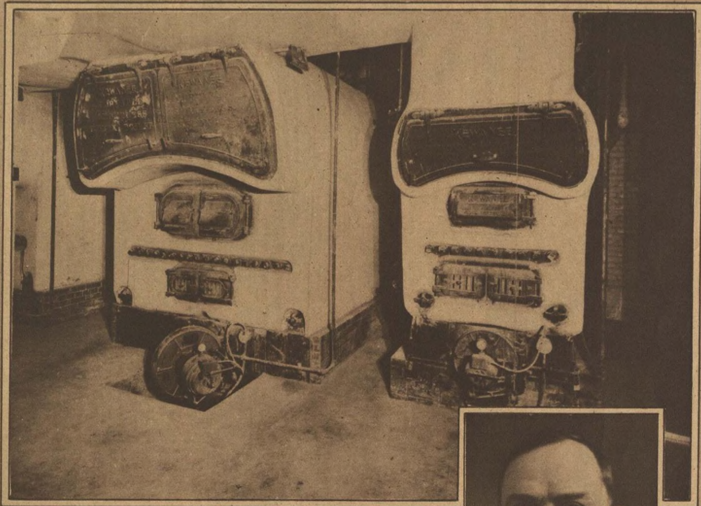
INTERIOR VIEW OF ENGINE ROOM
