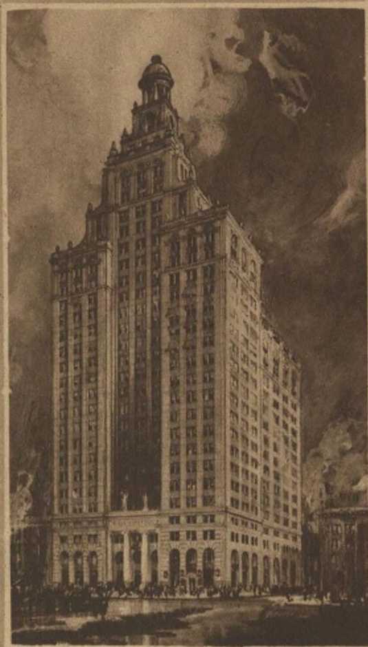
Niels Esperson Building of Houston, Texas. Equipped with Crane plumbing and heating materials throughout. Architect, John Ebersen, Chicago. General contractor, American Construction Co., Houston. Plumbing and heating contractor, Warren Co., Houston.
