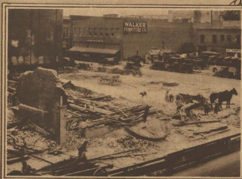
Clearing ground to prepare for excavation.
