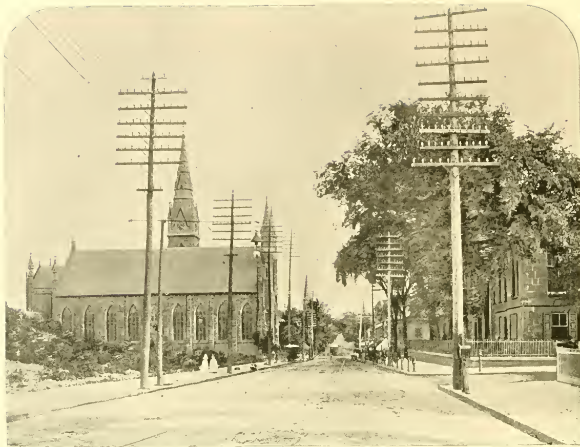
VIEW ON MAIN STREET, NEAR COURT HOUSE.
