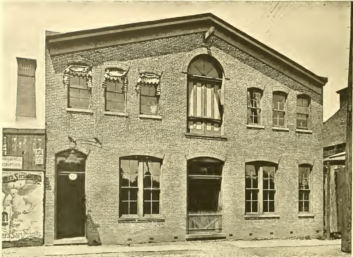
EXTERIOR OF THE PATERSON ELECTRIC LIGHT COMPANY'S WORKS.
