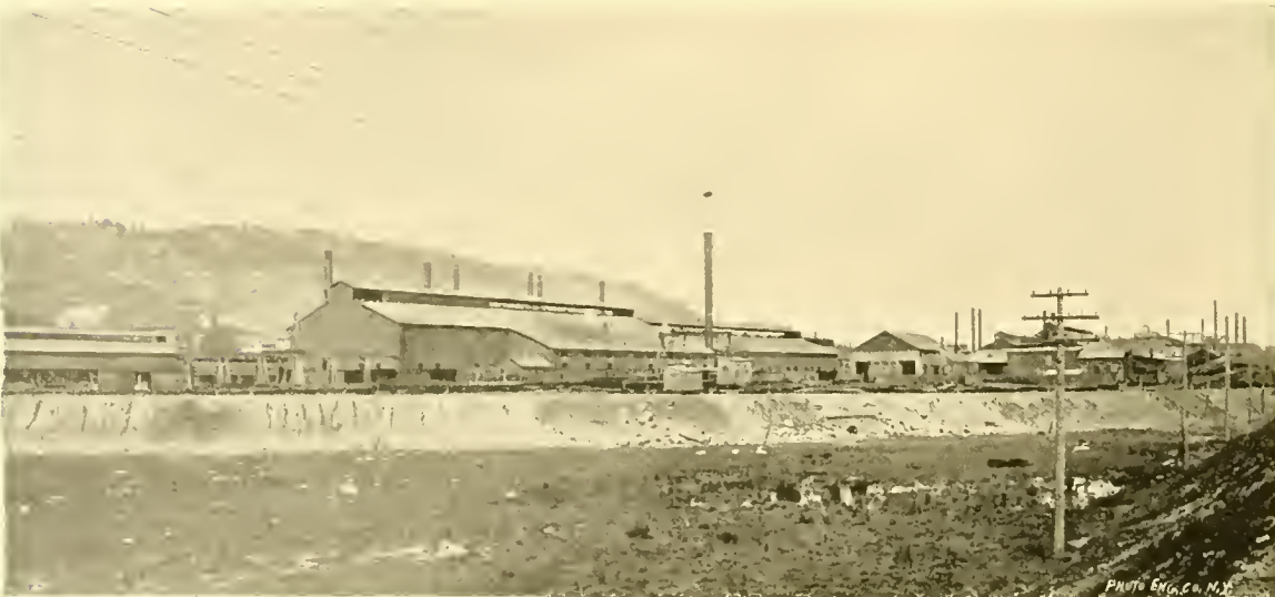
REAR VIEW OF THE PASSAIC ROLLING MILL COMPANY'S WORKS.
