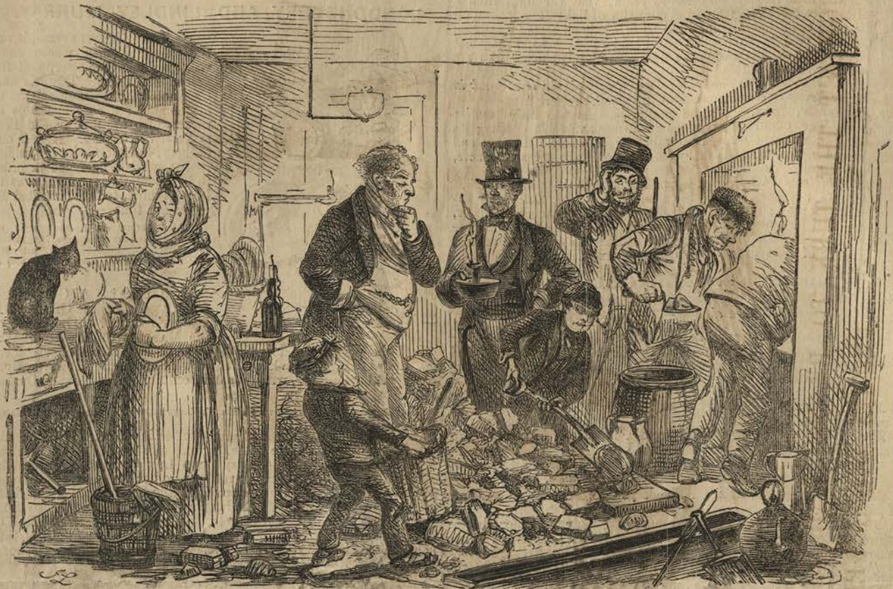
SOMETHING THE MATTER WITH THE KITCHEN BOILER.
