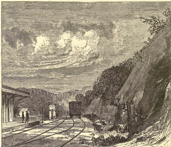
CUTTING ON THE SÃO PAULO RAILWAY, SHOWING DRIFT LYING ON DECOMPOSED ROCK.*
