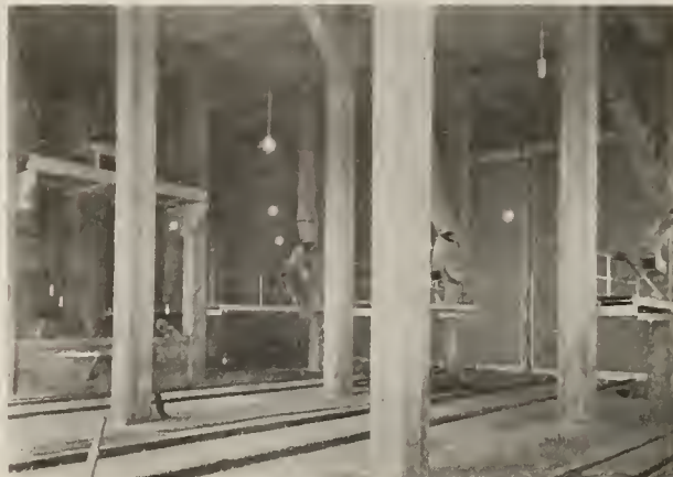
TRACK SHED, CARLOADING SPOUTS AND PLATFORMS
