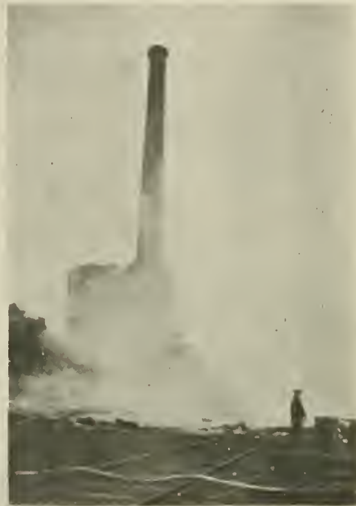
RUINS OF ELEVATOR "B" WITH POWER HOUSE WHICH PARTLY ESCAPED
