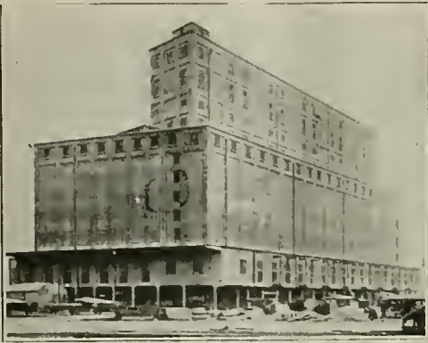
Manchester Ship Canal Elevator Manchester, England Capacity 1,500,000 Bushels Completed 1914
