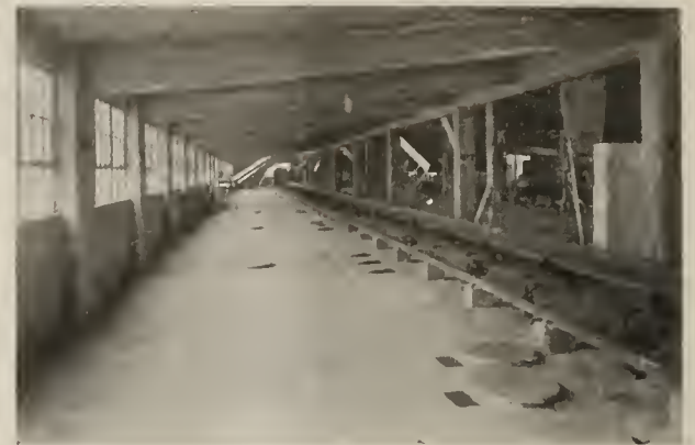
VIEW OF BIN FLOOR WITH CONVEYORS
