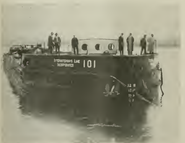
83,000-BUSHEL MOTOR SHIP ON N. Y. STATE CANAL
