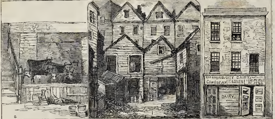
LONDON DEMOLITIONS; AND THE COW SHEDS.
