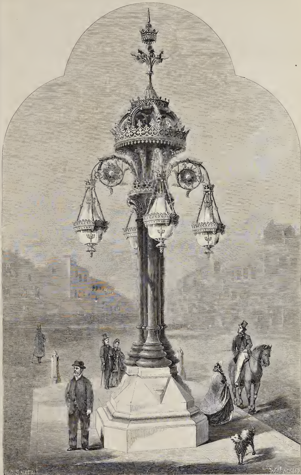
LAMP AND VENTILATING SHAFT ERECTED OVER THE SUBWAY, SOUTHWARK STREET, LONDON.
