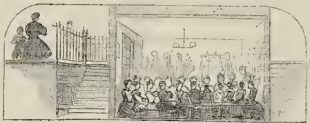
A Workshop: Making and Destroying.
