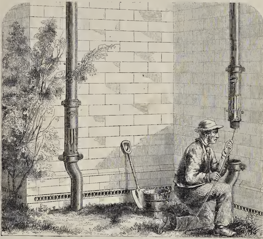
TELESCOPIC RAIN-WATER TUBES.
