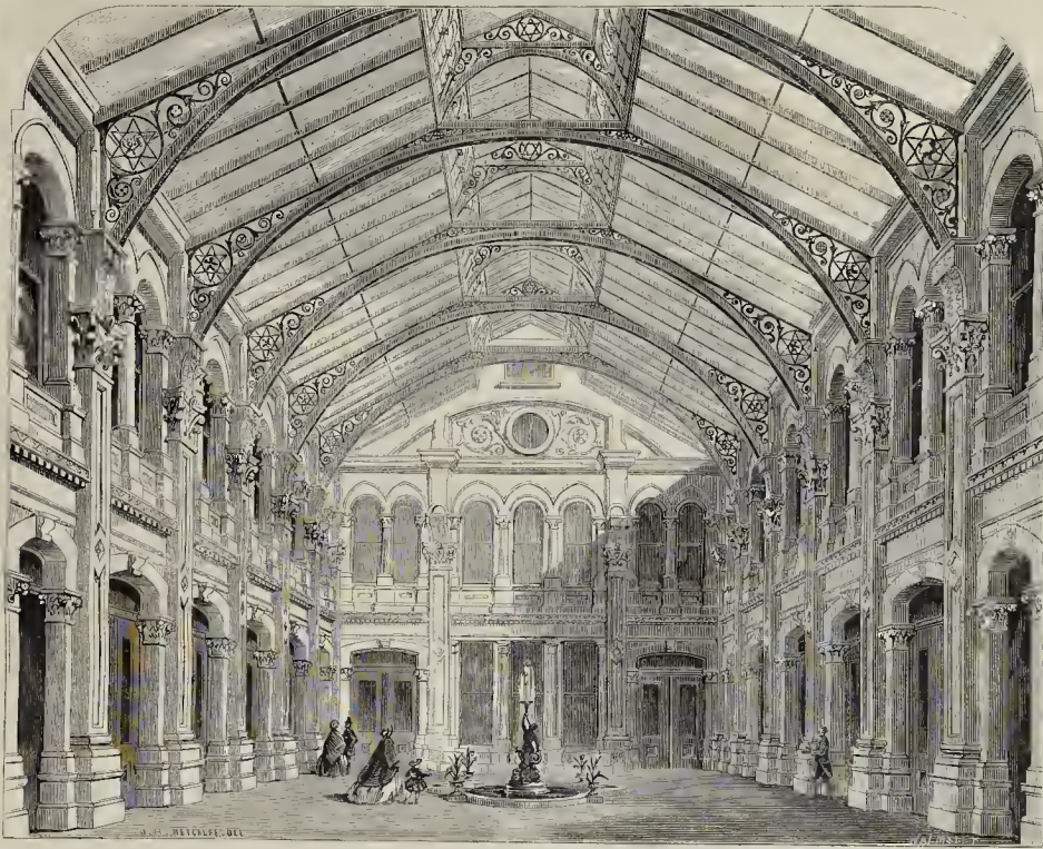
INNS OF COURT HOTEL, LONDON. VIEW OF THE INNER COURT.
