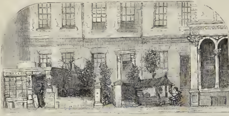
Building in advance.
