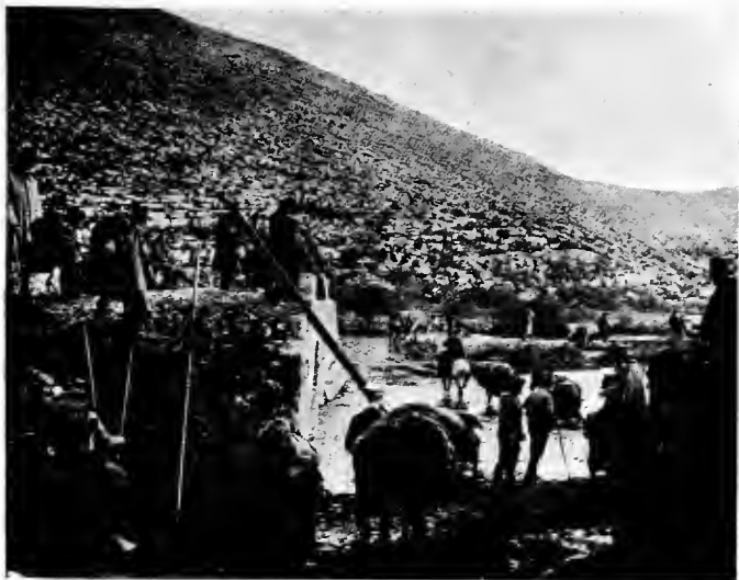
BROKEN BRIDGE AT FRONTIER BETWEEN MONTENEGRO AND ALBANIA
