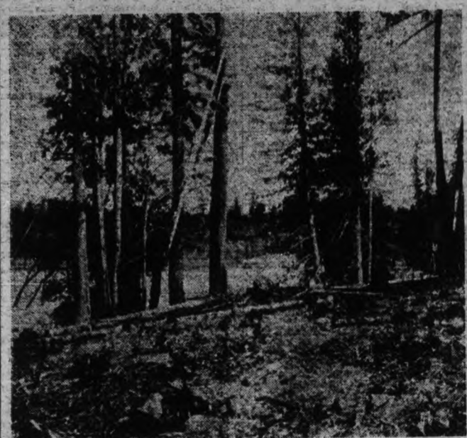
Much work has already been accomplished in clearing the 300 acres around Sooke Lake, which will be flooded when the level of lake is raised 15 feet.
