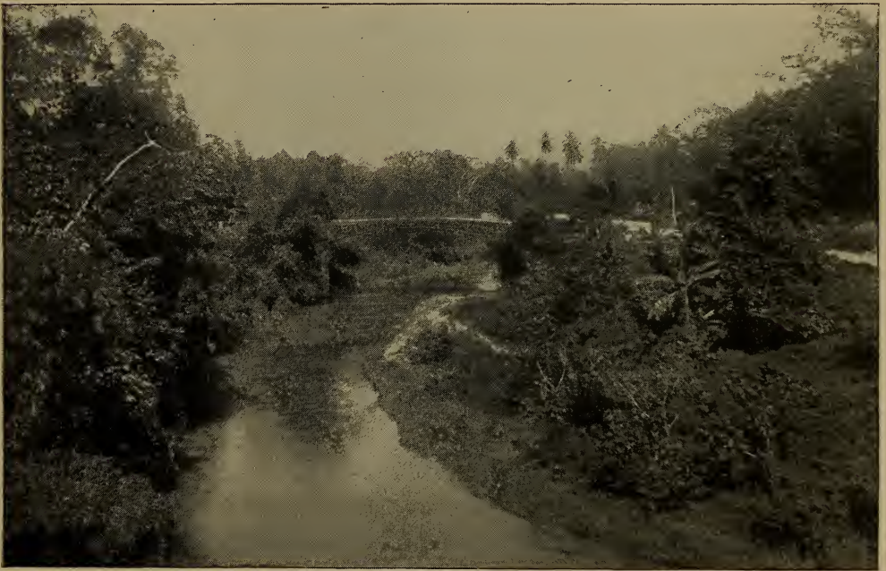
BRIDGE ON RIO COBRE RIVER.
