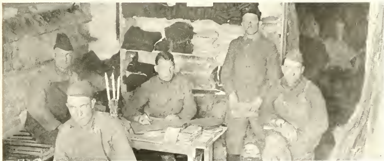
SUPPLY ROOM—COMPANY C.
