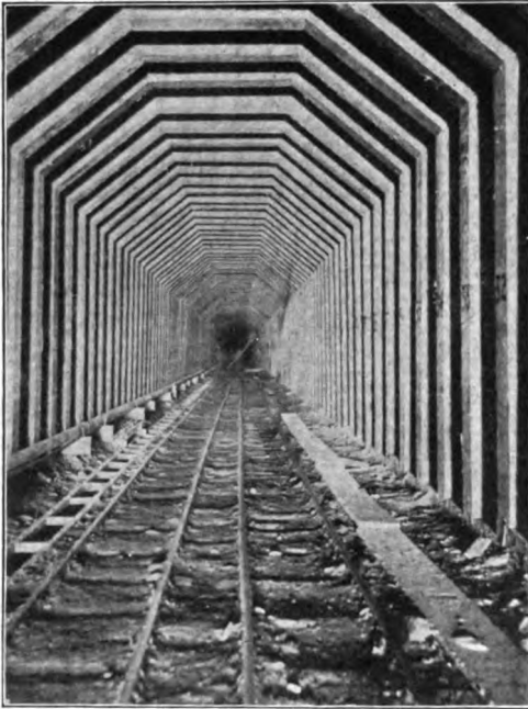
INSIDE VIEW OF WEST PORTAL OF GUNNISON TUNNEL,
