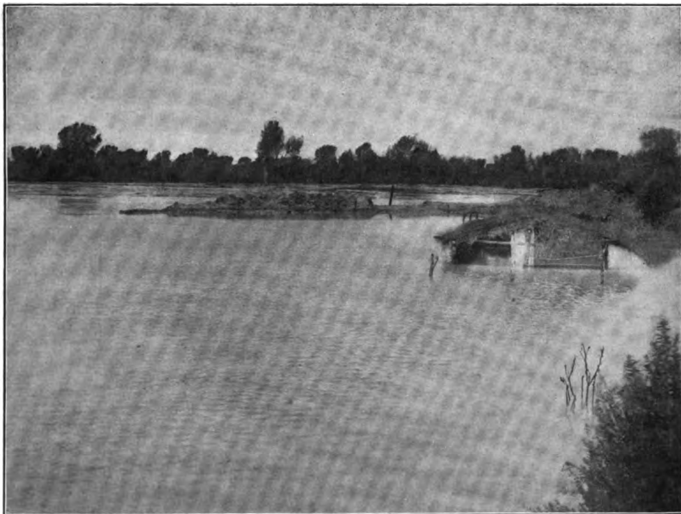
VIEW SHOWING THE FLOODED BANKS OF THE IMPERIAL HEADING No. 3, AT THE JUNCTION OF THE THREE HEADLANDS OF THE MAIN IMPERIAL CÁNAL, MEXICO, 1905.
