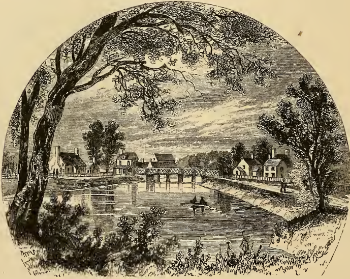
BRIDGE AT BLADENSBURG.
