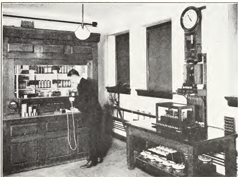
FIG. 63.— Automatic life tests of dry batteries
