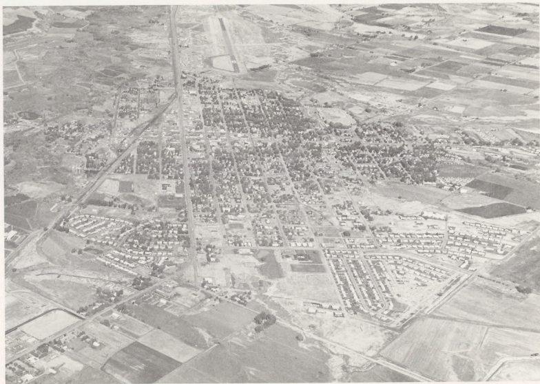
Figure B-17--An aerial view of Montrose, which faces critical water supply shortages.
