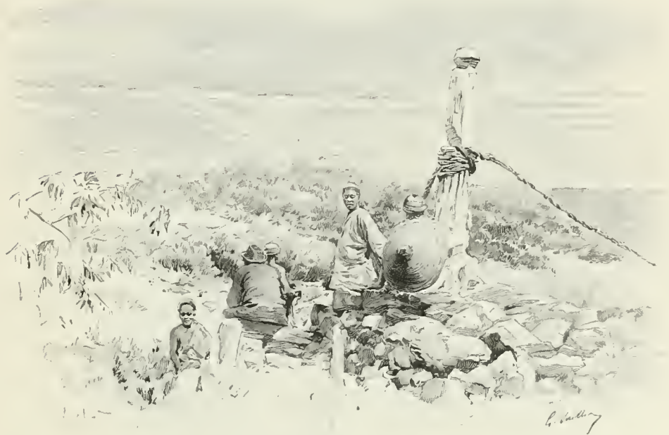
Attachment of Cord Bridge at Piao-tsen.
