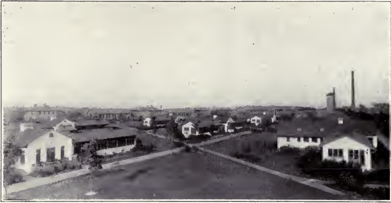
MUNICIPAL TUBERCULOSIS SANITARIUM North Crawford and Bryn Mawr Avenues View of Buildings from Southwest
