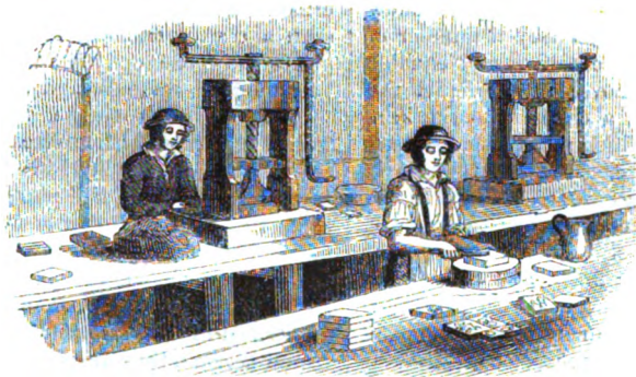
327. PRESSING AND SCRAPING TILES.
