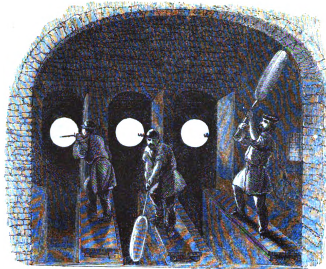
281. BLOWING AND SWINGING CYLINDER GLASS.
