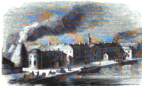
331. WEDGWOOD'S FACTORY AT ETRURIA, IN STAFFORDSHIRE.
