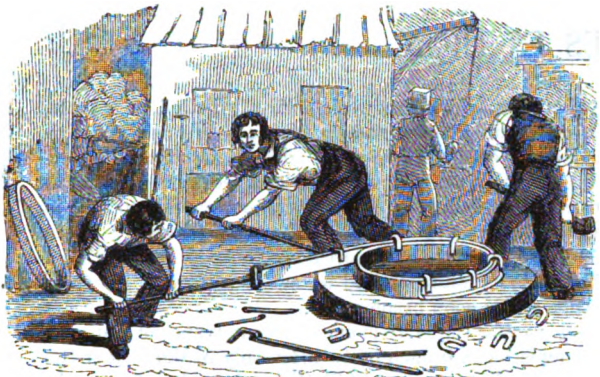
422. BENDING THE TIRE FOR RAILWAY-CARRIAGE WHEEL.
