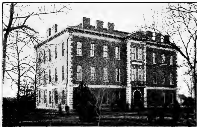
Main Building, Central Wesleyan College, Warrenton, Mo.
