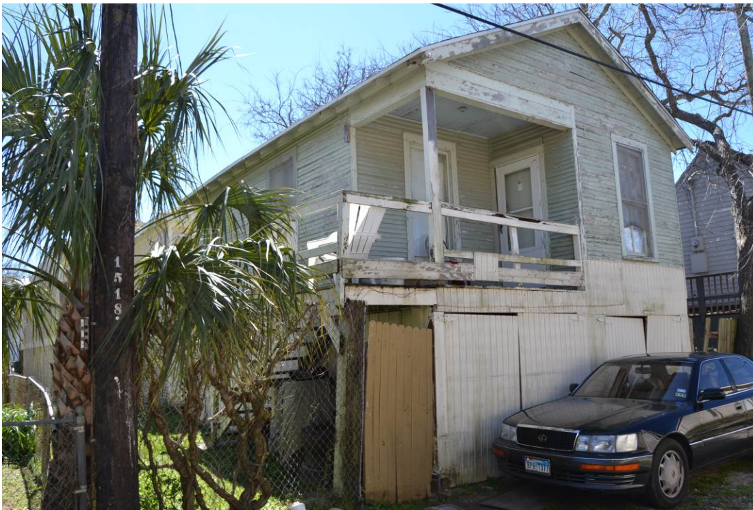
Photo No. 37. Oblique view of alley house at 1524 Avenue L (RID 689273b). View facing southwest. February 2016.
