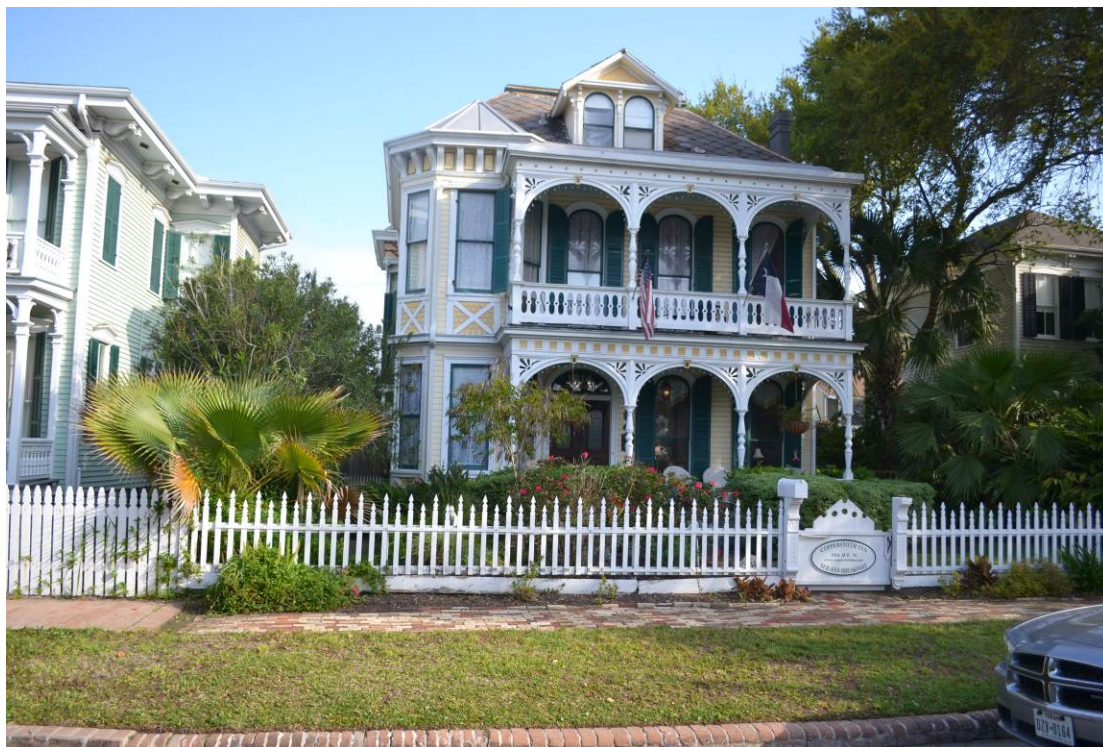
Photo No. 28. Façade of 1914 Avenue M (RID 61a). View facing north. April 2015.
