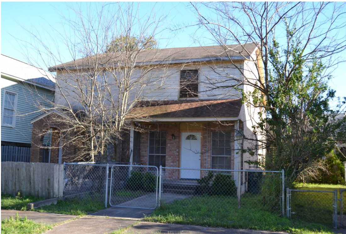
Photo No. 18. Oblique view of 1509 Avenue L (RID 683545). View facing southeast. February 2016.
