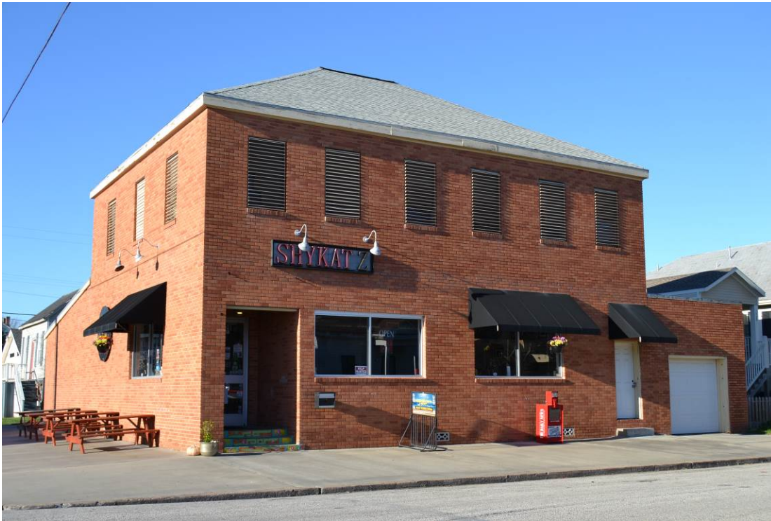
Photo No. 36. Oblique view of 1528 Avenue L (RID 689274a). View facing northeast. February 2016.
