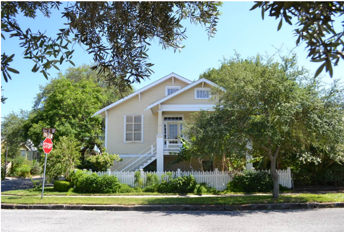
Photo No. 14. Façade of 1701 Avenue K (RID 689301). View facing south. April 2015.
