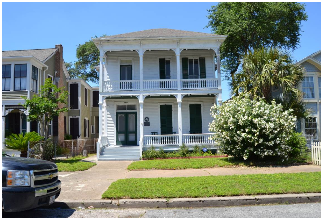
Photo No. 8. Façade of 1808 Avenue K (RID 689547). View facing north. April 2015.
