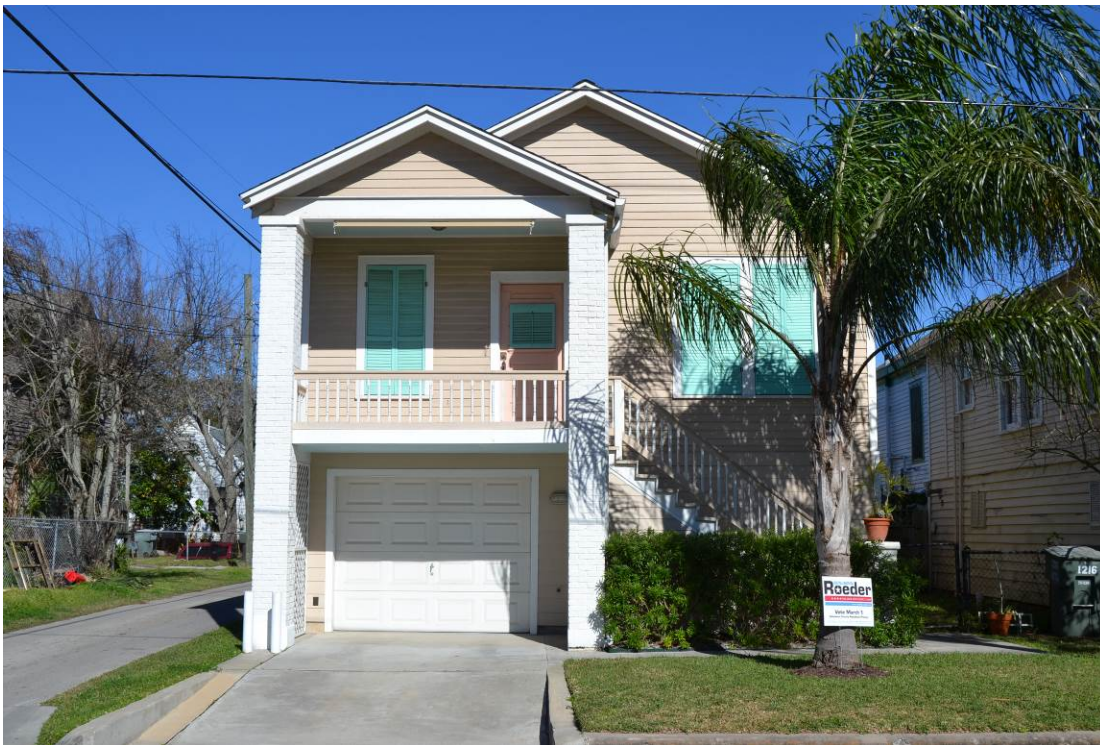
Photo No. 33. Façade of 1214 16th Street (RID 6851285). View facing east. February 2016.
