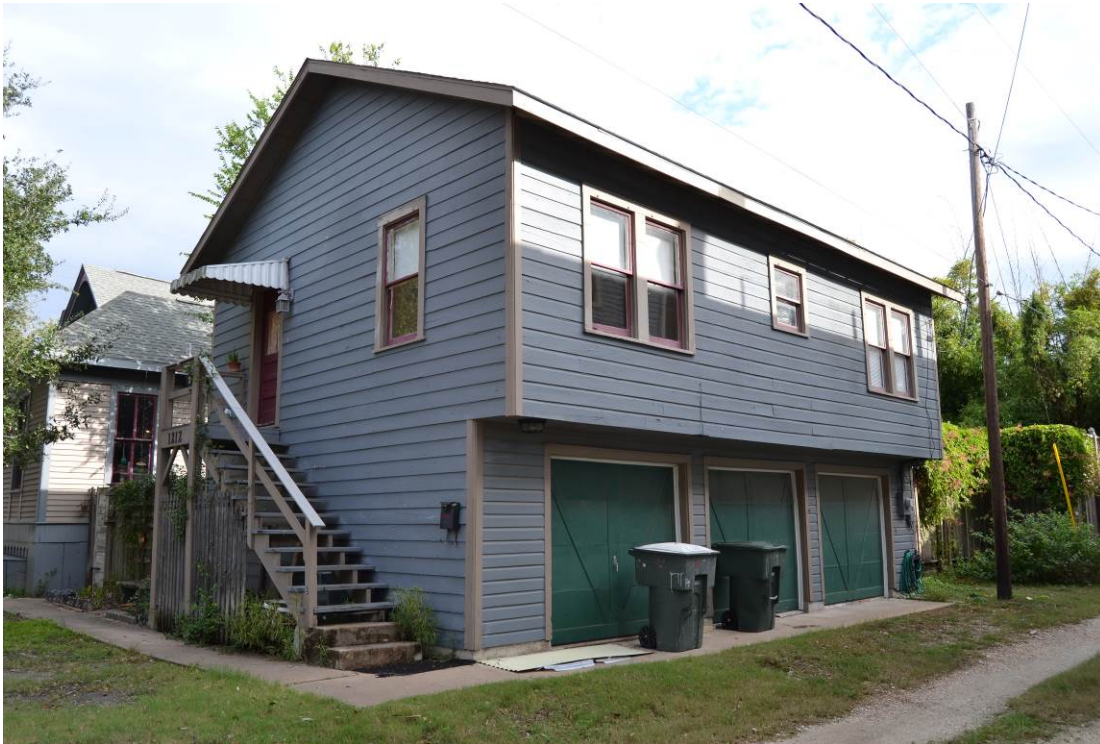
Photo No. 15. Oblique view of an alley house at 1925 Avenue L (RID 52b). View facing northeast. November 2015.
