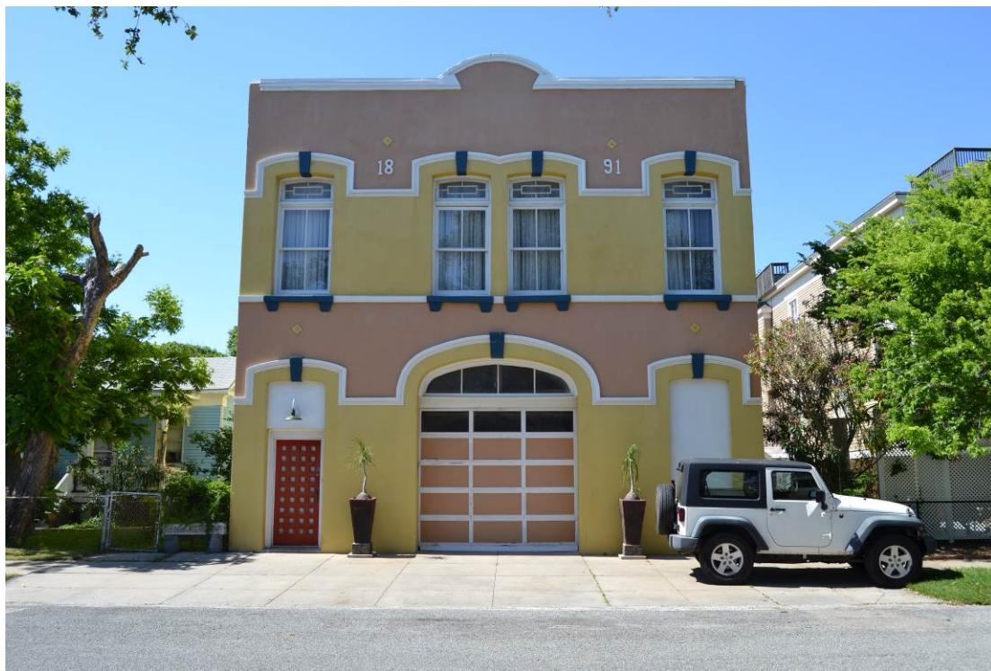
Photo No. 35. Façade of 1614 Avenue K (RID 689523). View facing north. April 2015.
