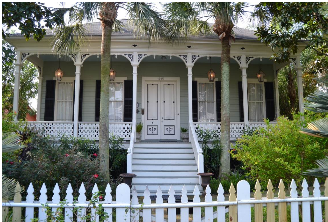
Photo No. 26. Façade of 1915 Avenue M (RID 688138). View facing south. April 2015.
