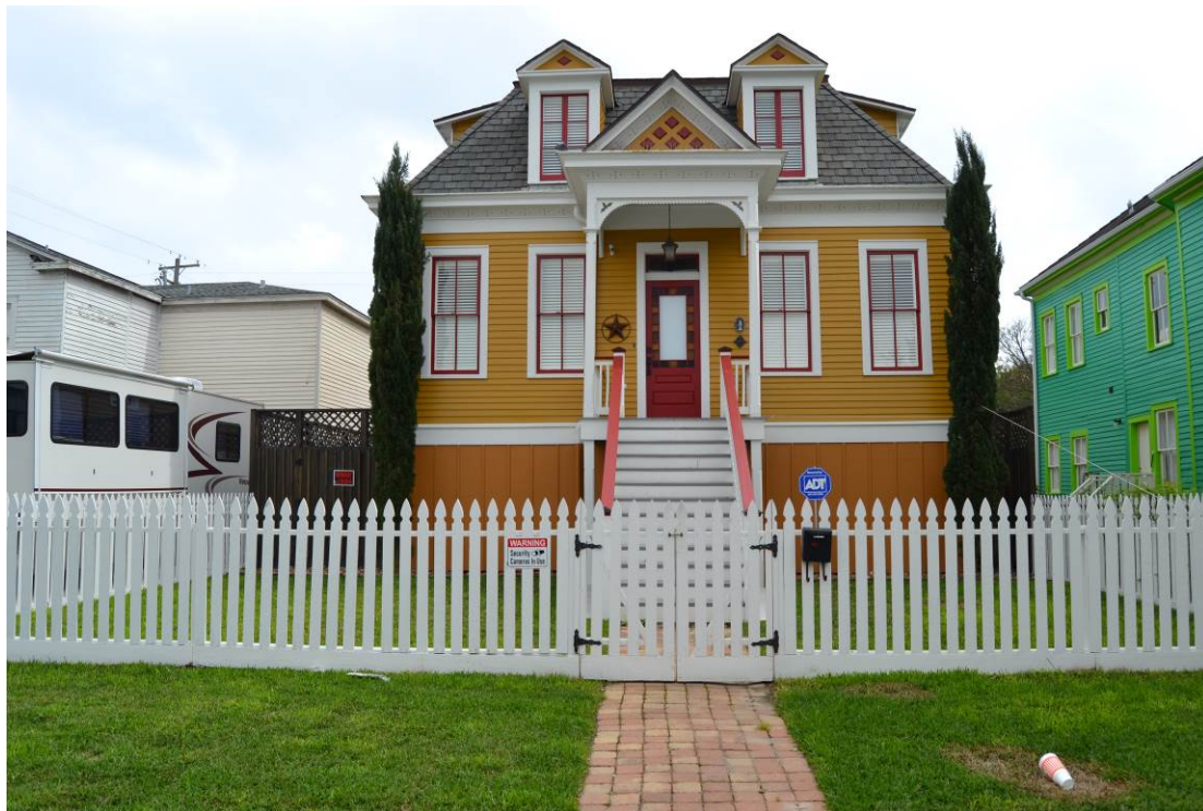
Photo No. 7. Façade of 1905 Avenue M½ (RID 688198). View facing south. April 2015.
