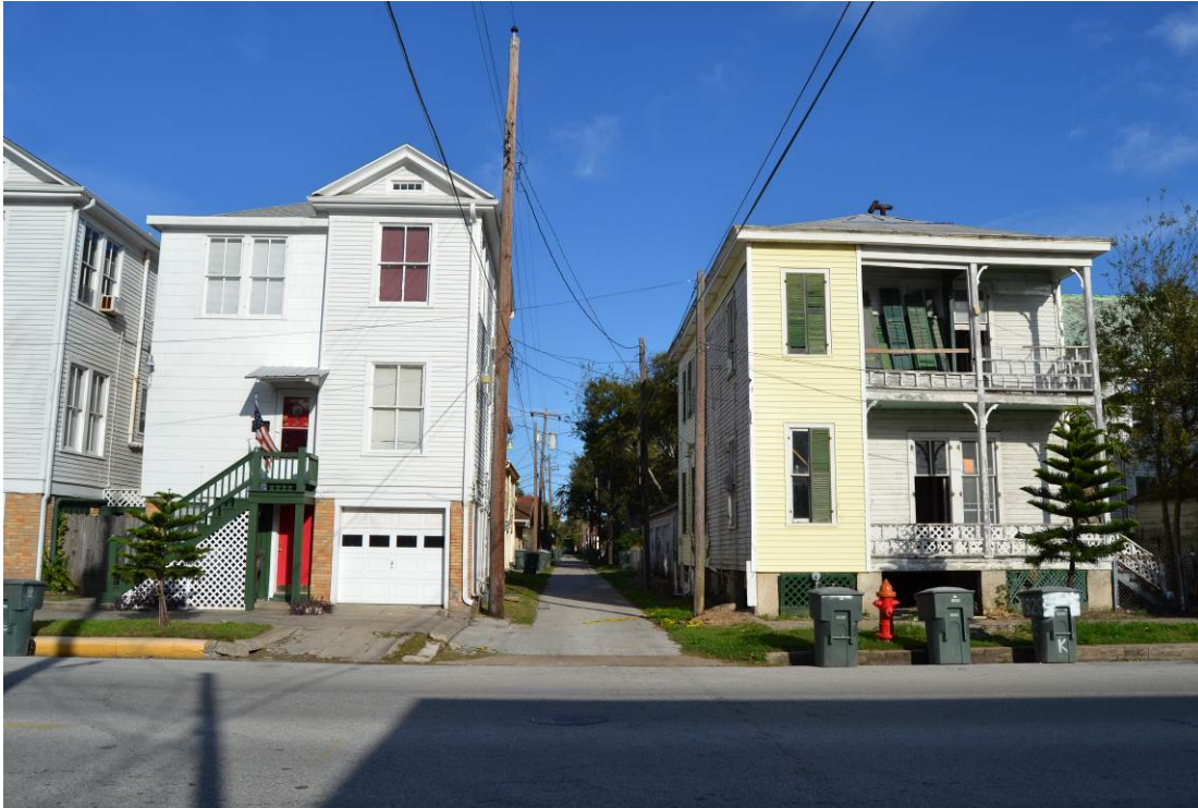
Photo No. 17. Contextual view of powerlines at alley between Broadway Street and Avenue K. View facing east. November 2015.
