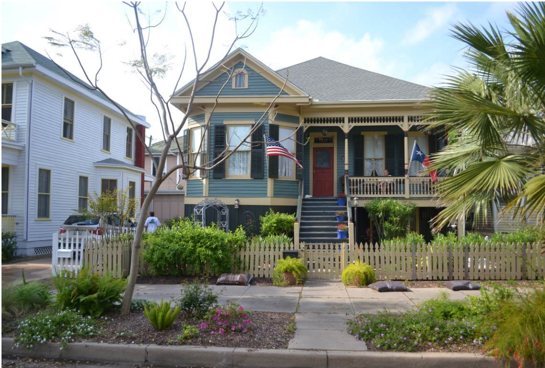
Photo No. 9. Façade of 2024 Avenue M (RID 48a). View facing north. April 2015.
