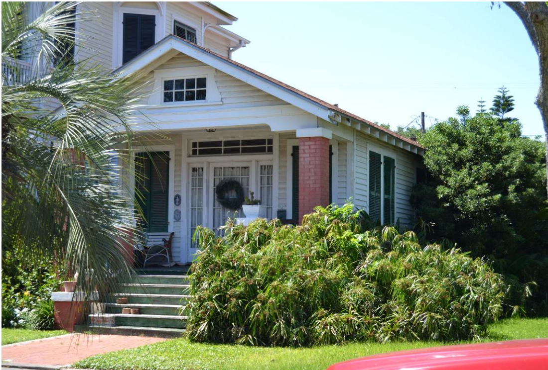
Photo No. 32. Oblique view of 1714 Avenue K (RID 698533). View facing northwest. April 2015.
