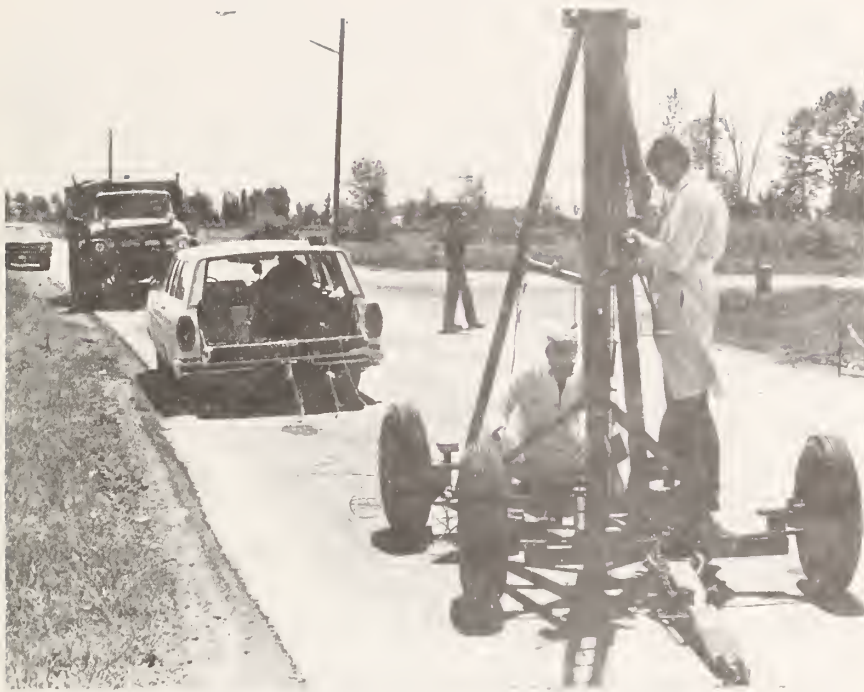
Figure B.24 CAL impulse generator
