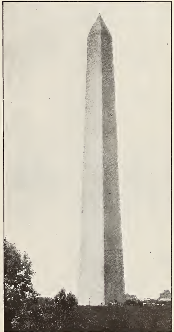
Washington monument around which tests of the direction of radio waves were made. The natural wave length of the monument was found to be about 800 meters
