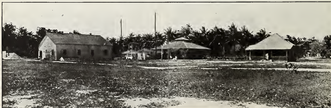
THE RADIO STATION AT SANTA MARTA, COLOMBIA Showing the power house, operating house, and residence for employees
