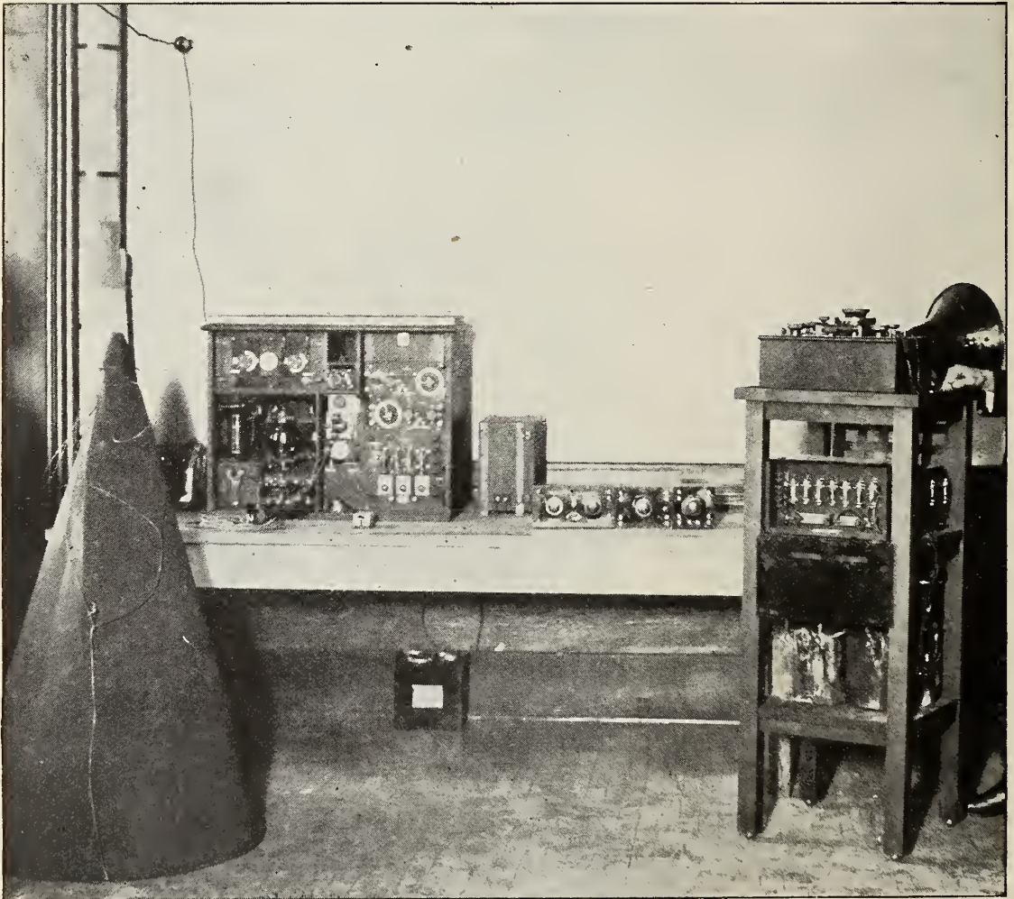
THE INTERIOR OF THE EDMONTON JOURNAL'S BROADCASTING STATION
