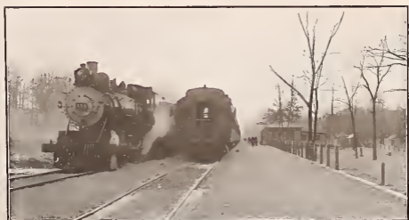
KANSAS CITY & SOUTHERN RAILWAY DEPOT, SULPHUR SPRINGS, ARKANSAS
