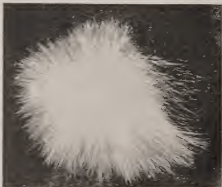
IMPRESSION OF AN ELECTRIC SPARK ON A PHOTOGRAPHIC PLATE.
