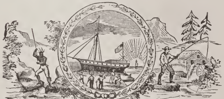
COAT-OF-ARMS OF NEW HAMPSHIRE.
