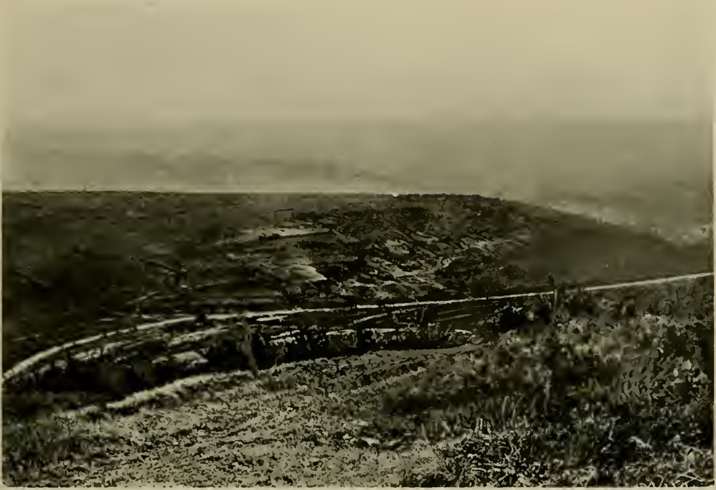
THE ROAD FROM LES EPARGES TO TRESAUVAX
