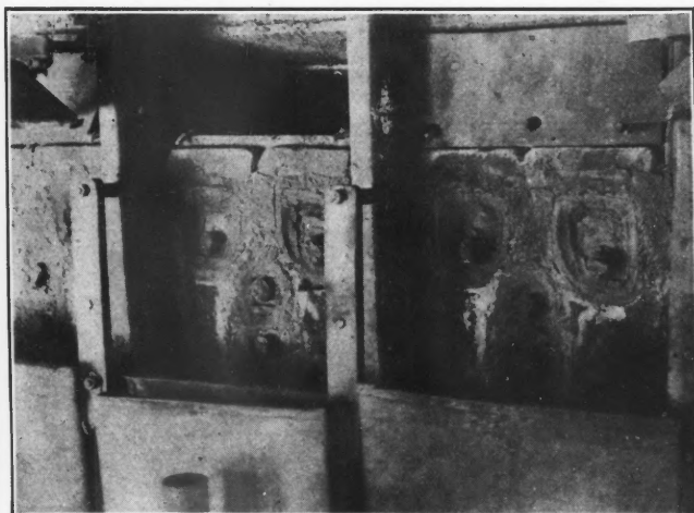
FIG. 2. DIRECT-FIRED FURNACE AT WALTER CRONECKHUTTE, SHOWING DAGNER CONDENSERS
