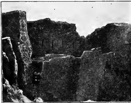
Loopholes through Which Arrows Were Shot.
