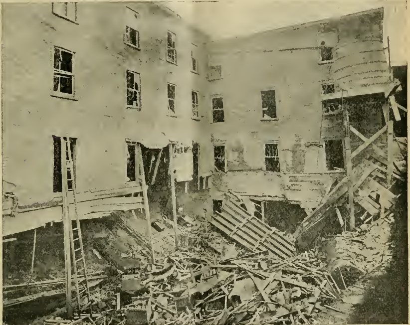
RUIN WROUGHT BY THE EXPLOSION OF A HORIZONTAL TUBULAR BOILER.
