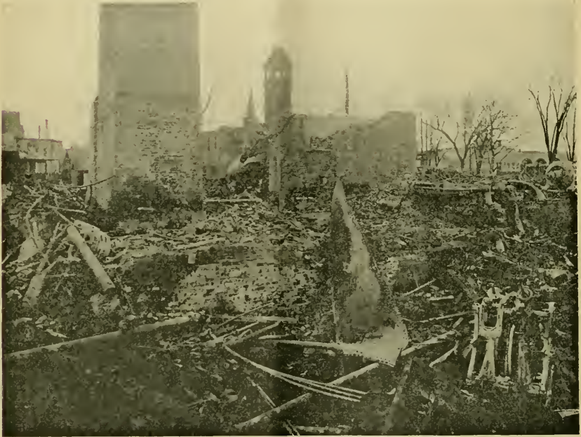
FIG. 5.—GENERAL VIEW OF THE FACTORY RUINS.
