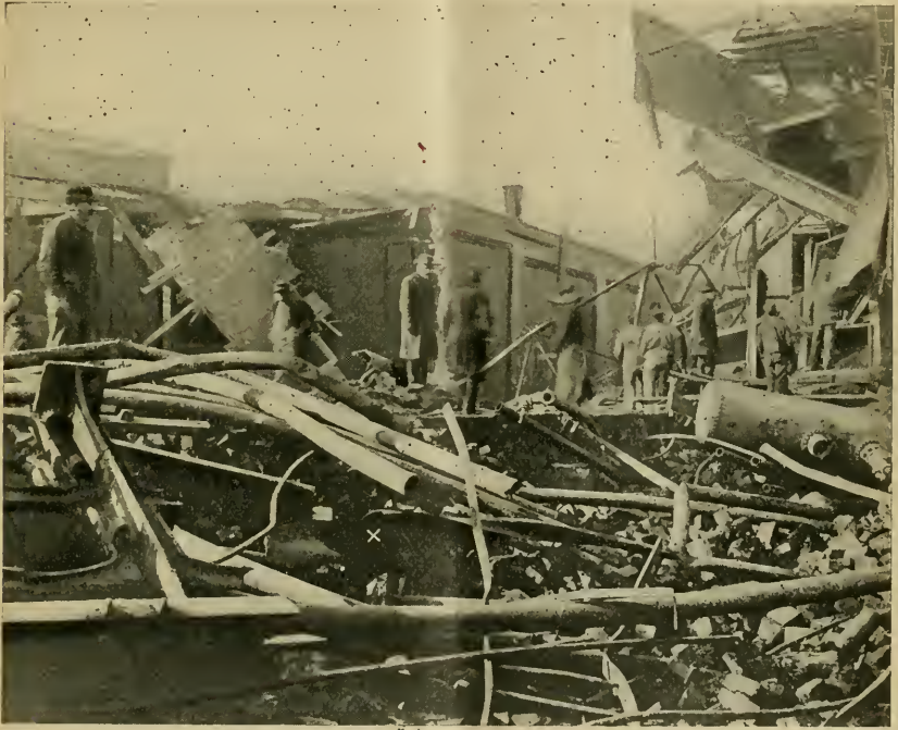
FIG. 3. — SHOWING THE BURSTED TUBE. (SEE THE WHITE CROSS.)
