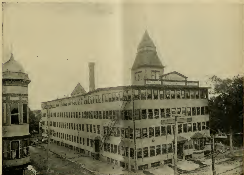
FIG. 1.—THE R. B. GROVER COMPANY PLANT BEFORE THE EXPLOSION.
