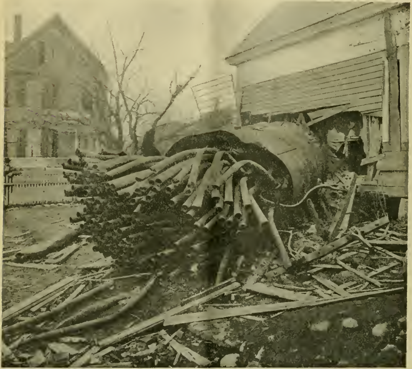
FIG. 9.—SHOWING THE BOILER IN ITS FINAL POSITION, AGAINST THE HOOD HOUSE.
