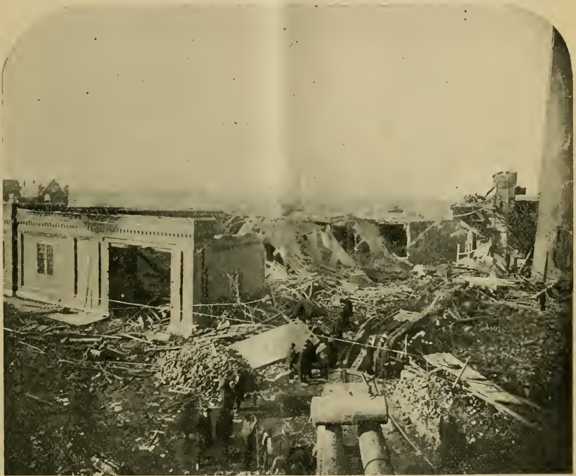
FIG. 5. — GENERAL VIEW, SHOWING BOILER NO. 7 IN THE FOREGROUND.
