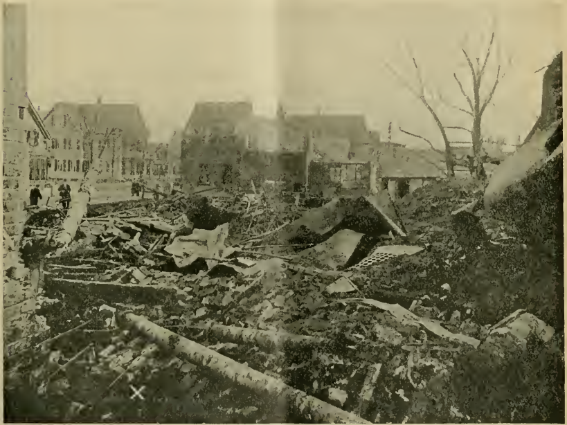
FIG. 6.—VIEW OF THE FACTORY RUINS, LOOKING TOWARD ENGINEER ROCKWELL'S HOUSE.
