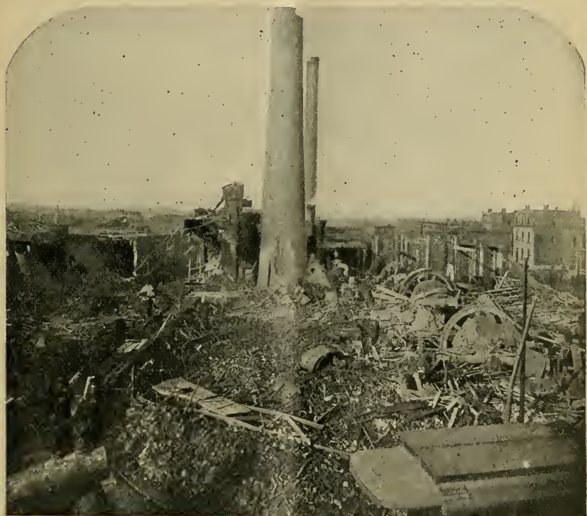
FIG. 1. — GENERAL VIEW OF THE RUINED PLANT.
