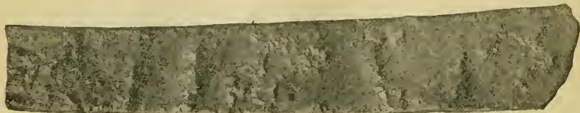
FIG. 2.—A PIECE CUT FROM THE SHELL PLATES, SHOWING CORROSION.
