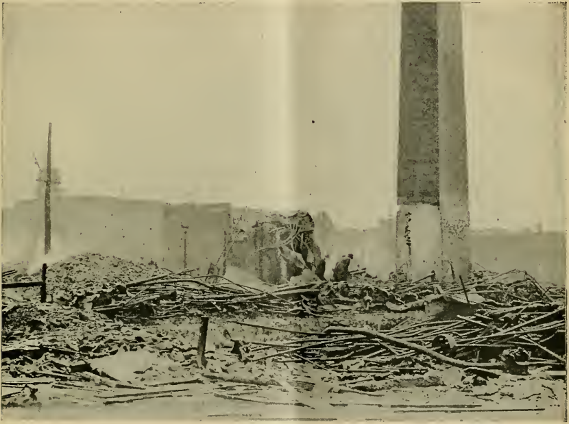
FIG. 4.—GENERAL VIEW OF THE FACTORY RUINS.
