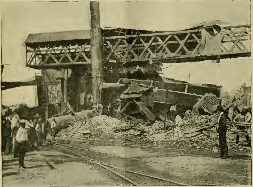
FIG. 1. — GENERAL VIEW OF RUINS.
