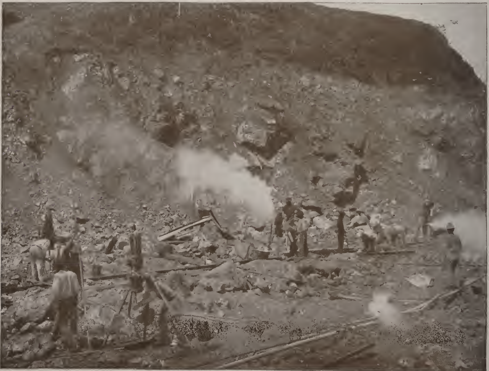
Steam Drills at Work in Bas Obispo Cut DIGGING THE PANAMA CANAL
