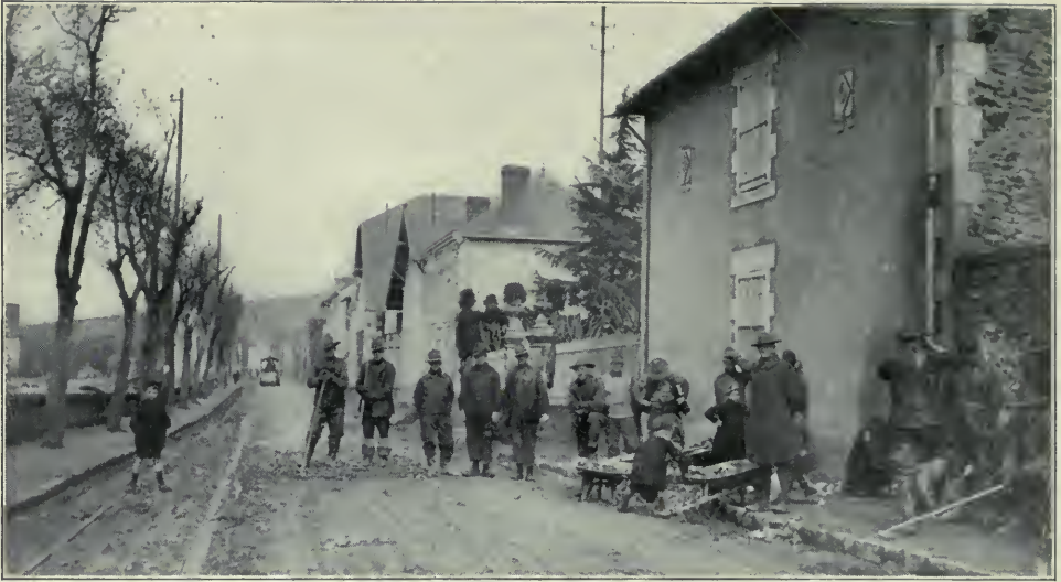
ENGINEERS RE-SURFACING ROAD IN AIX, HAUTE VIENNE
