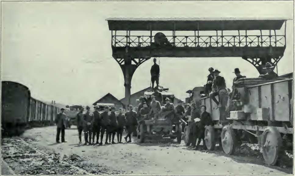
COMPANY B, 311TH ENGINEERS, UNLOADING ROCK
