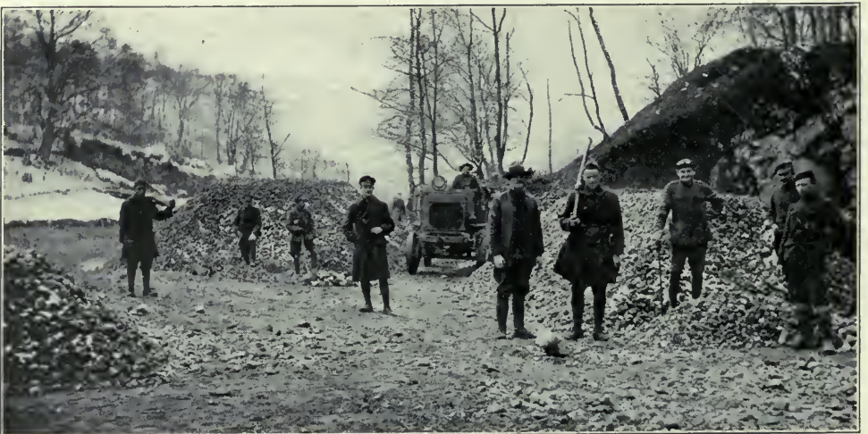
GERMAN PRISONERS WORKING FOR 311TH ENGINEERS AT LA COURTINE
