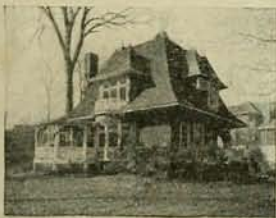
A No. C-24x IDEAL Boiler and 555 ft. of 38-in. AMERICAN Radiators, costing the owner $250, were used to Hot-Water heat this cottage.
