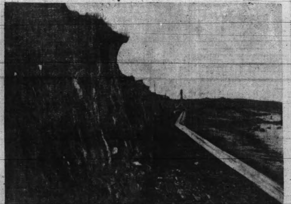
WASTING OF DALLAS ROAD FORESHORE.
