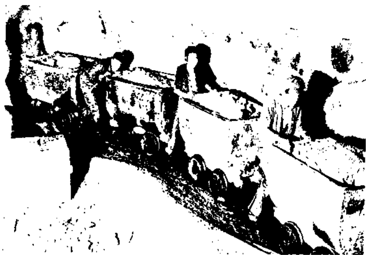
TRUCKING THE ORE TO THE SHAFT
