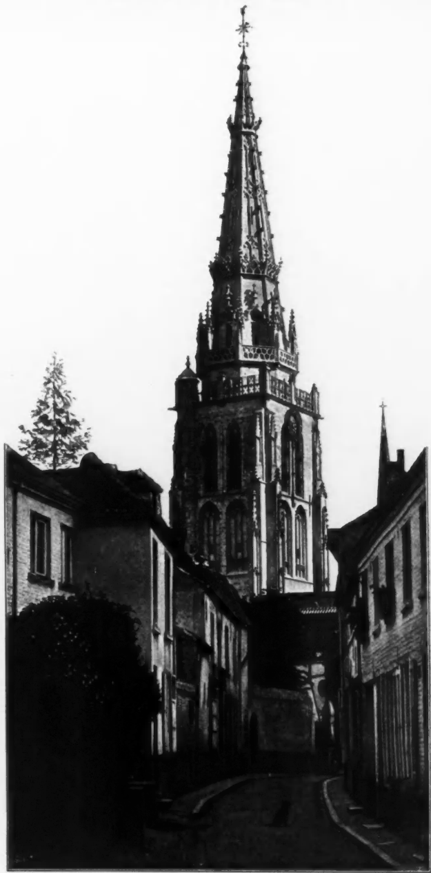
Stone Spire added to the Tower of the Church of Saint Pierre, Anderlecht, J. J. VAN YSENDYCK, Hon. Corr. Mem. R. I. B. A., Architect, Brussels.
