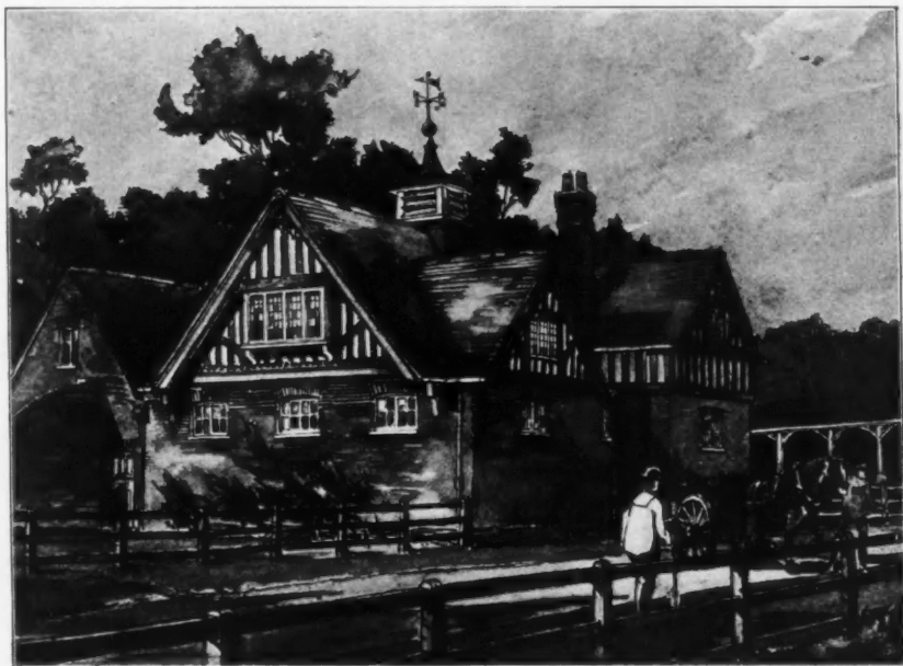
1704. Stables, Matfield, Kent , EDGAR S. UNDERWOOD, Architect.
