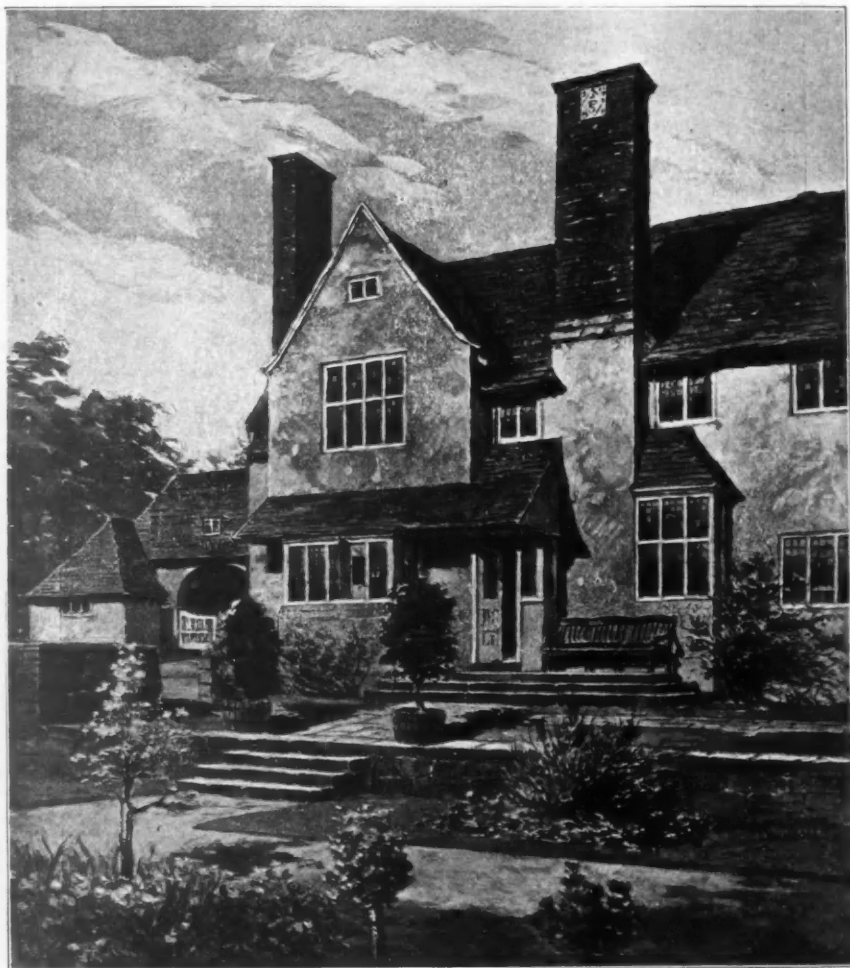
1644. Corner of House, Edgbaston, Birmingham, BATEMAN AND BATEMAN, Architects. (For Plans, see p. 45.)
