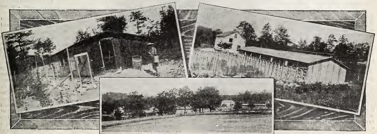
In the group of illustrations above are given several views of the Sands & Beilman poultry farm, Hawley, Pa. In the lower picture a general view of the main buildings is to be had, on the right is the brooder house and incubator cellar, while on the left is shown one of the laying houses. This house is 110 x 15 feet, contains five pens in which a total of 405 birds were kept during the last year. The average egg production was 148 eggs per capita from the birds confined in this house.
