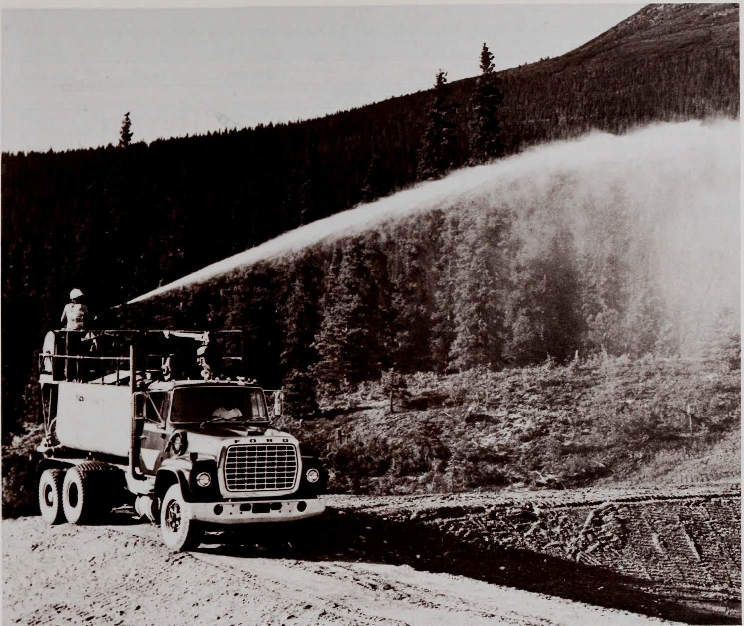
Revegetation is part of the rehabilitation of disturbed areas. Here, hydroseeding is used to spread a mixture of water, grass seed, and mulch to prevent erosion along the trans-Alaska pipeline. (Atlantic Richfield Company)
