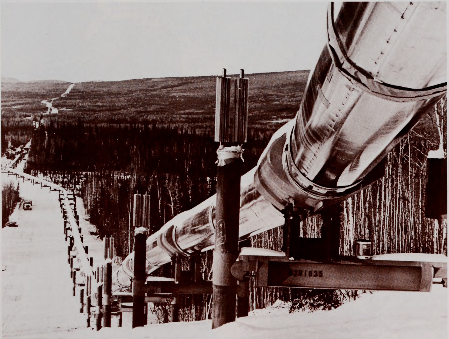
The trans-Alaska pipeline spans 800 miles and crosses three major mountain ranges. (Alyeska Pipeline Service Company)
