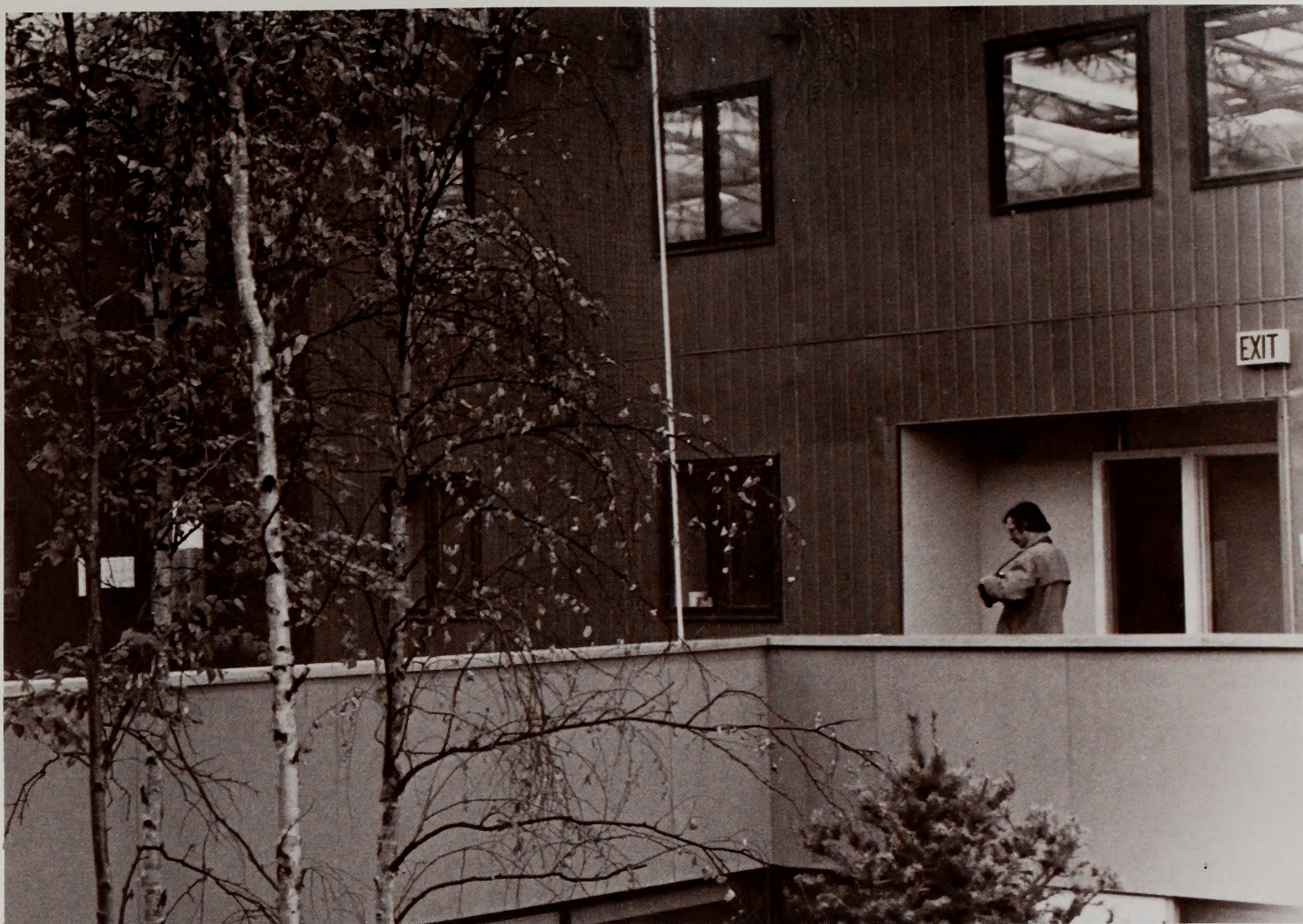
The SOHIO-BP and Atlantic Richfield camp facilities at Prudhoe Bay represent the highest "state of the arts" in arctic construction. The only birch trees north of the Brooks range are housed in the SOHIO-BP base camp. (Mary Aho, AEIDC)
