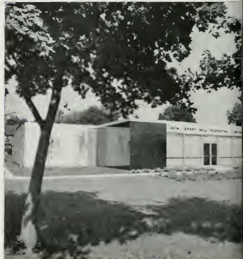
New Jersey Bell Telephone Co. building in Succasunna where ESS office is located.
