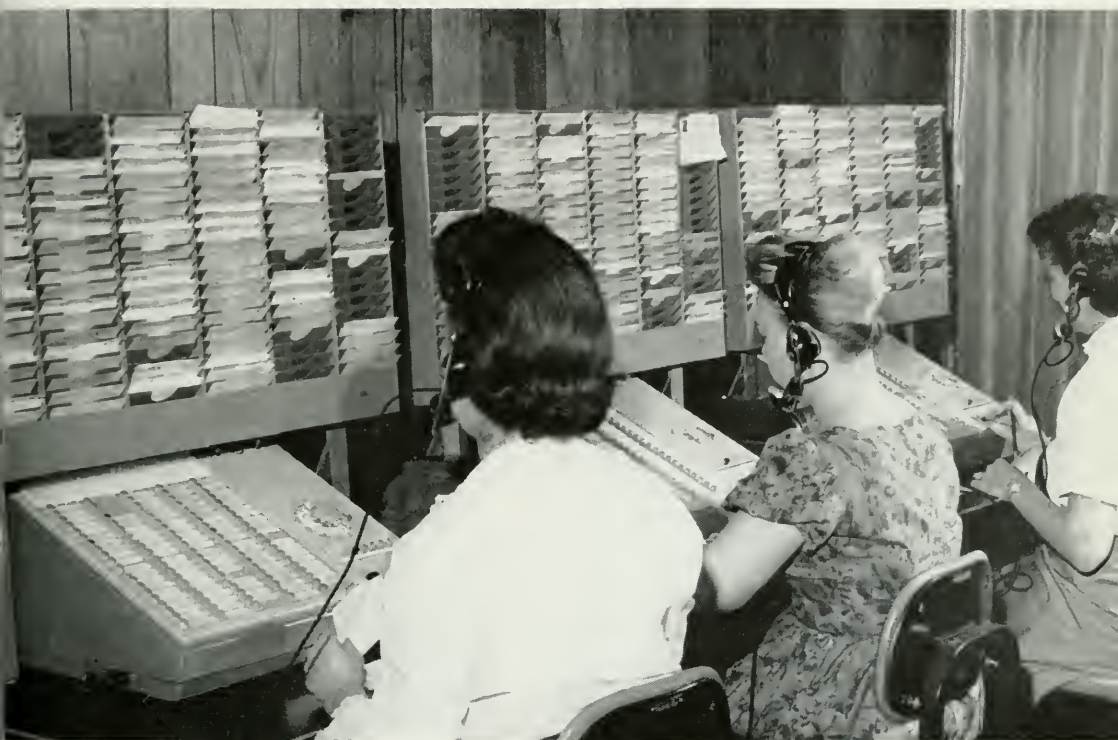
The 1A Telephone Answering System in trial installation: a quiet, pleasant place to work. The new, compact consoles are easier to use and more attractive than present equipment.
