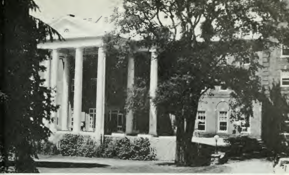
The main entrance of the Otesage Hotel in Cooperstown, N. Y., where the Bell System's Data Communications Training Program is located.
