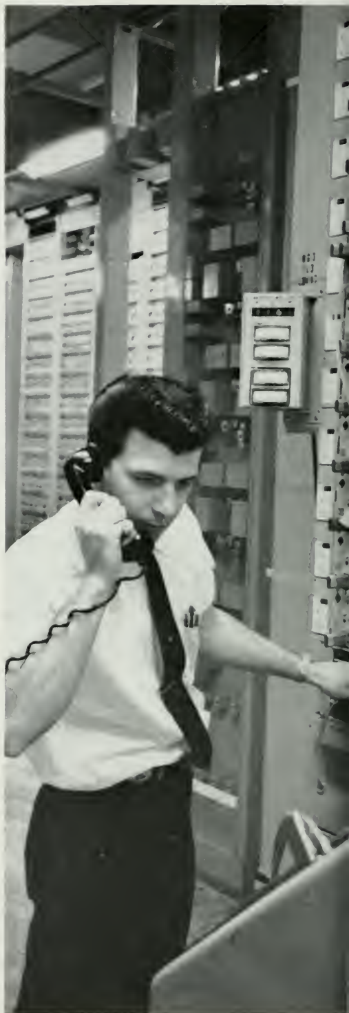
Transistorized terminal equipment is seen above; craftsman checks transmission levels of a group of broadband circuits.
