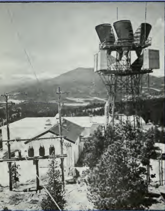
Microwave site on Buckhorn Mountain, Colo. is one of Bell System's highest. Below: wave breakers are assembled to protect wave guide equipment on a mountain top microwave tower.
