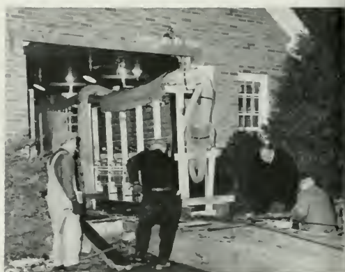
Top. Hole was cut in wall of Antioch, Ill. central office to remove 28-position board. Below. Huge board on its way with escort; sign reads: "emergency switchboard for fire stricken Richmond, Ind. from Illinois Bell."
