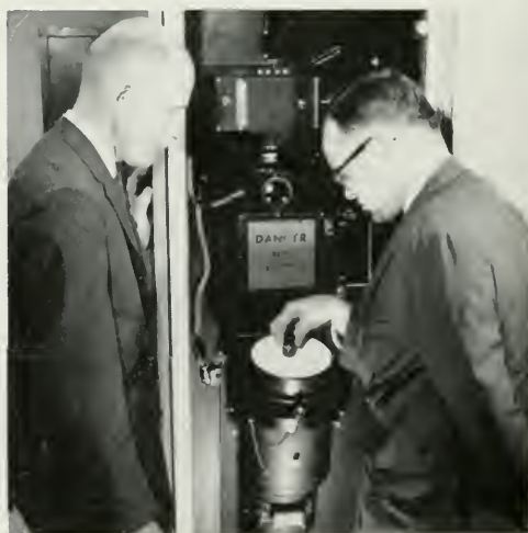
Overhead camera photographs letters generated on screen of this cathode ray tube.
