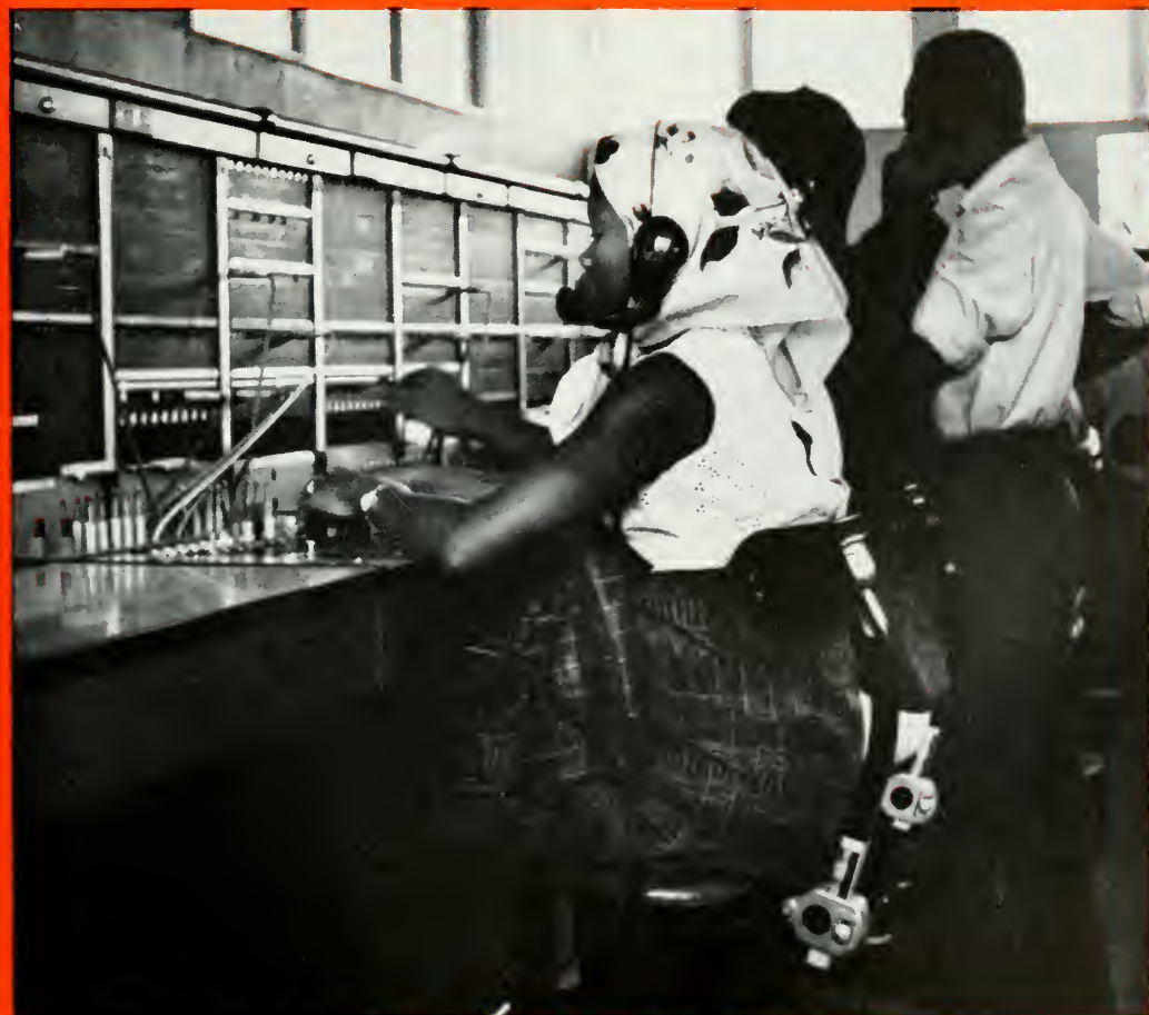
Typical operating room at Kaduna in the Northern Region.
