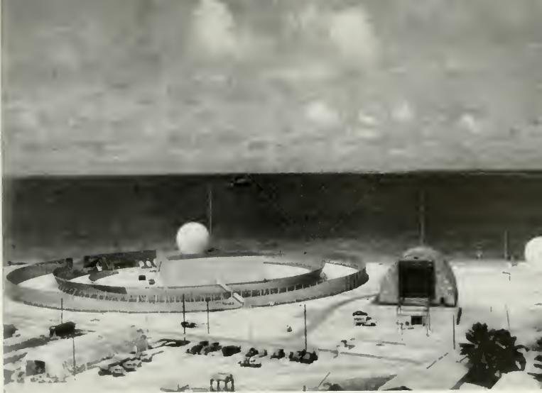
Discrimination Radar antenna, at left, on Kwajalein in South Pacific, used by Army in anti-missile-missile tests.
