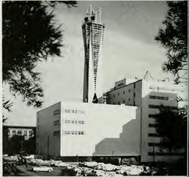
Microwave towers in downtown locations pose particular problems. Towers shown here—top right, Bartlesville, Okla. (Southwestern Bell); lower right, Los Angeles (Pacific Telephone); left, Seattle (Pacific Northwest Bell)—are each examples of attractive, individual solutions which harmonize with both their building and locale.
