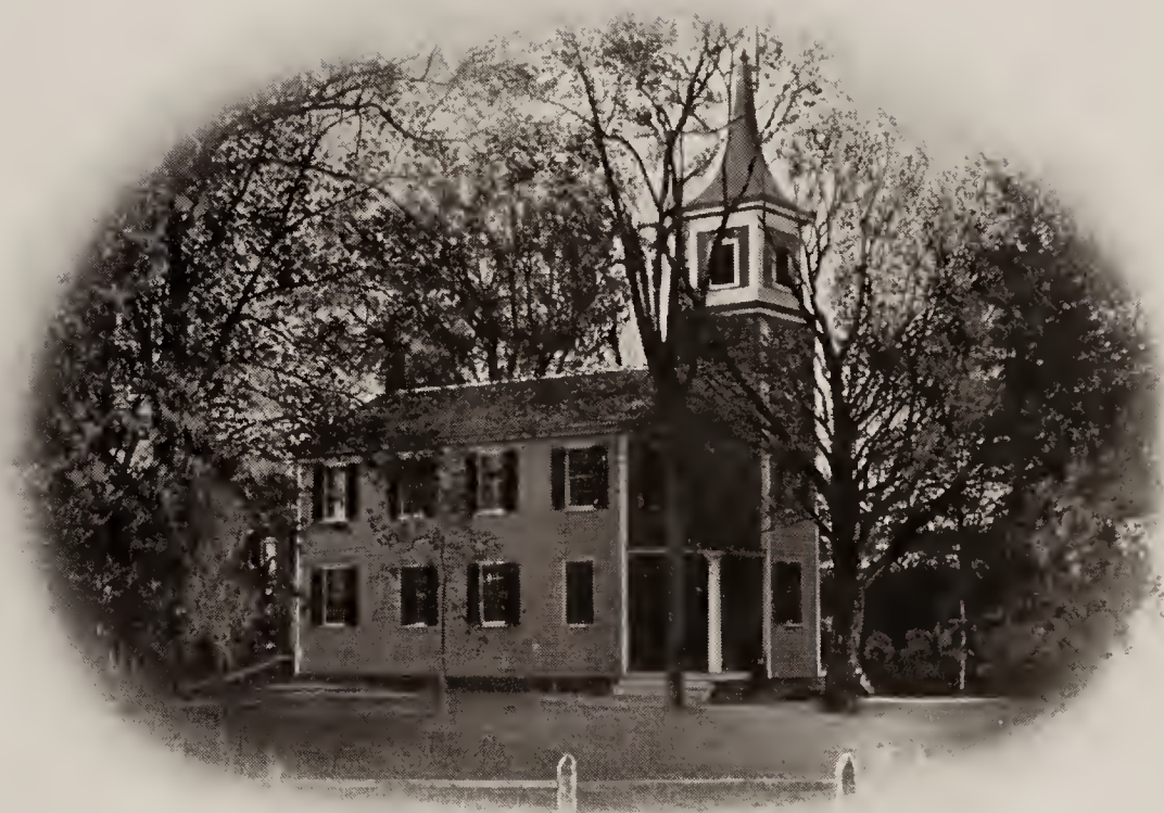
OLD SCHOOL BUILDING
